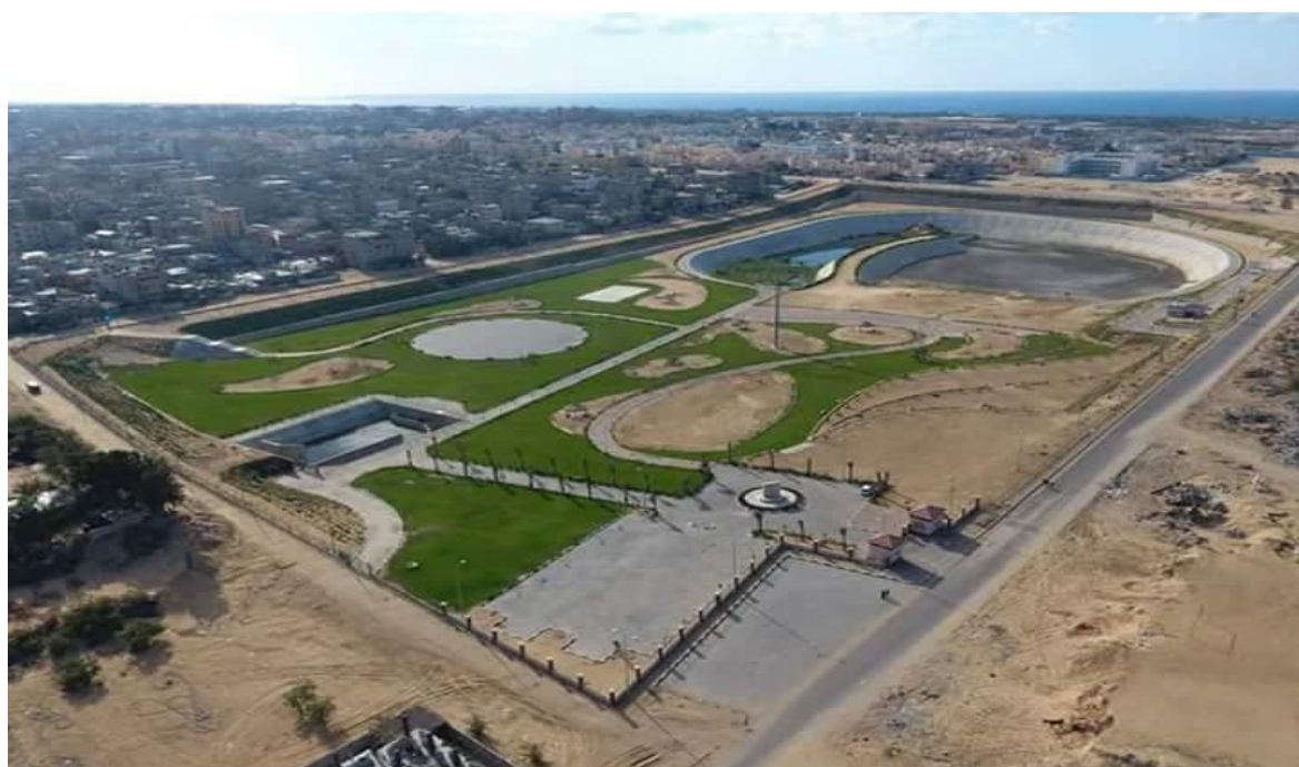
Al Amal Lagoon (After the intervention)
