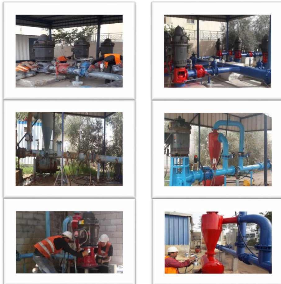
Figure 8: Water facilities Repair, Refurbishment and Rehabilitation Works
