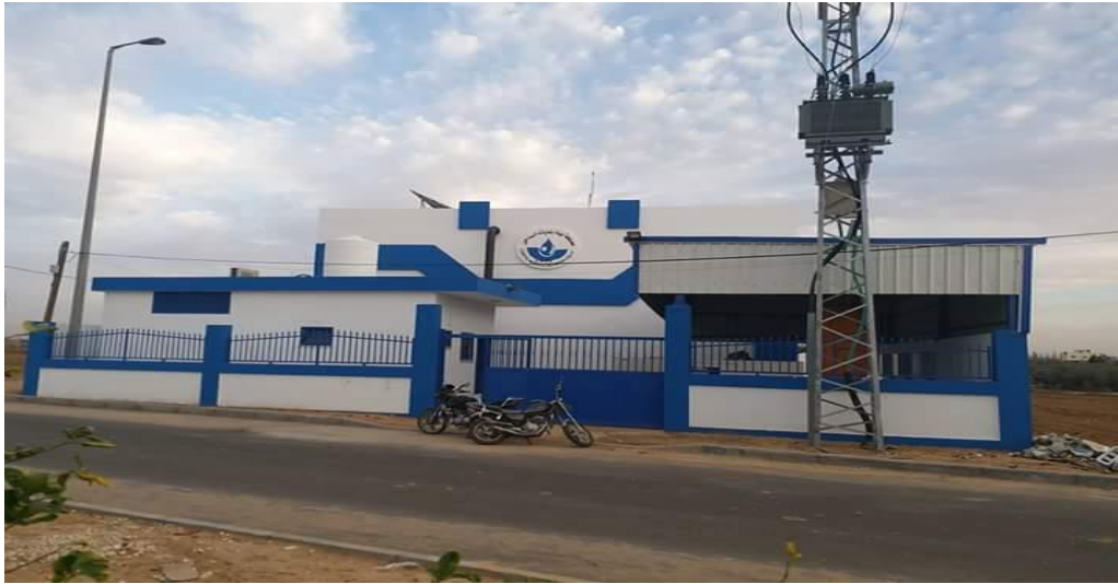
Figure 20: Abasan Water tank
