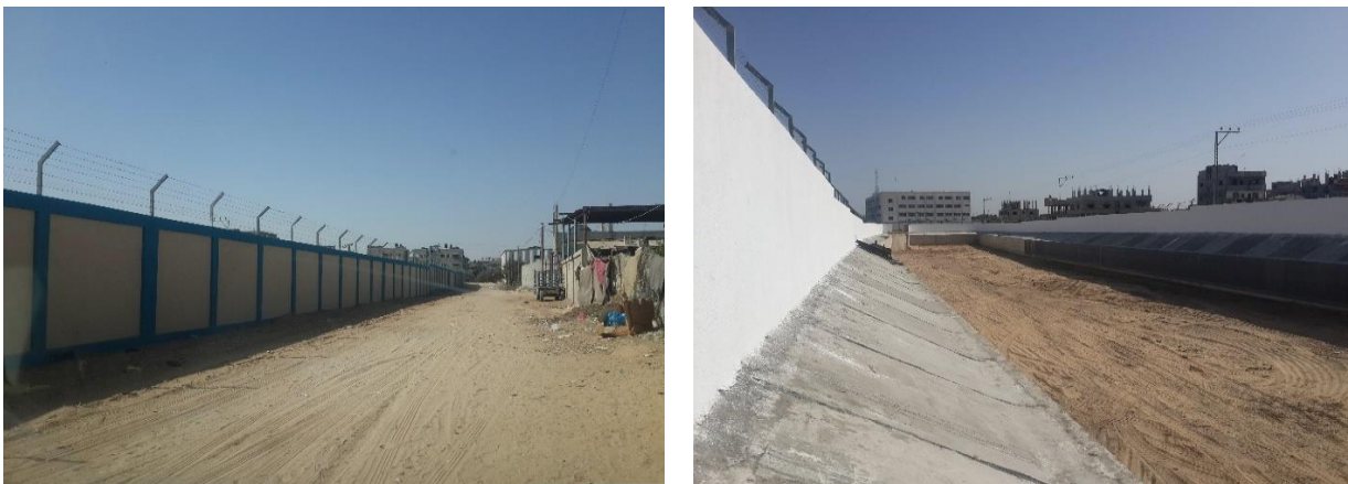
Figure 29: Boundary wall of Al Junina Storm water Pond
