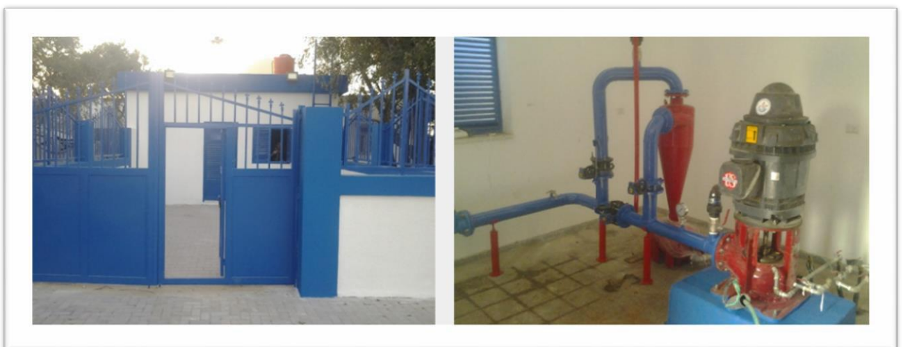
Figure 5: Al Mosadar water well
