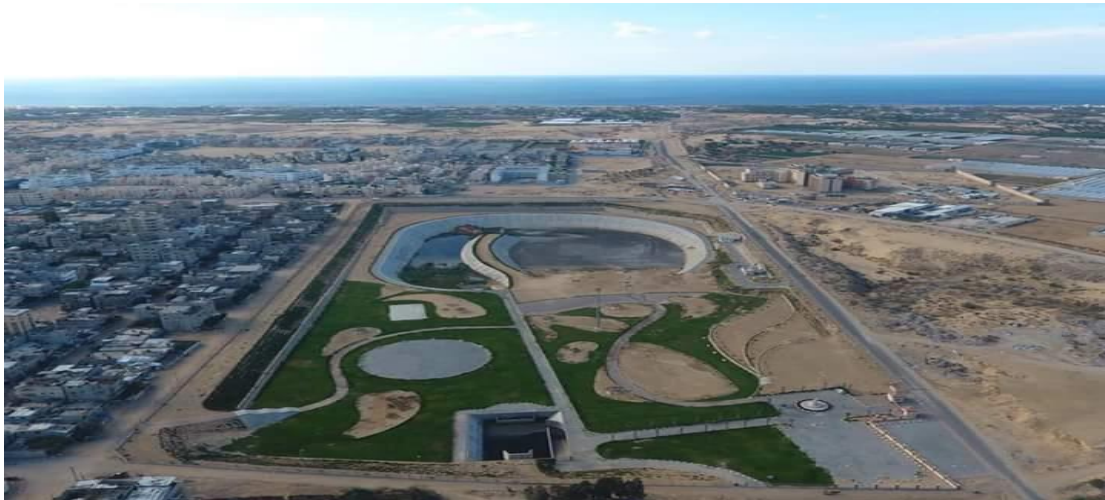
Figure 28: Al Amal Storm Water Project
