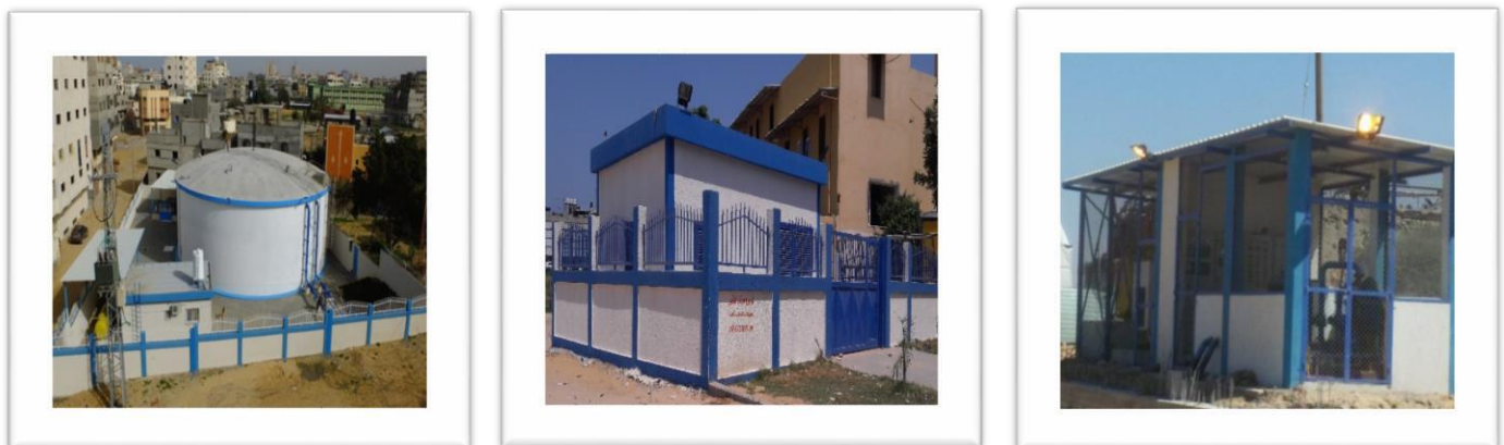
Figure 24: KFW Reconstruction Activities
