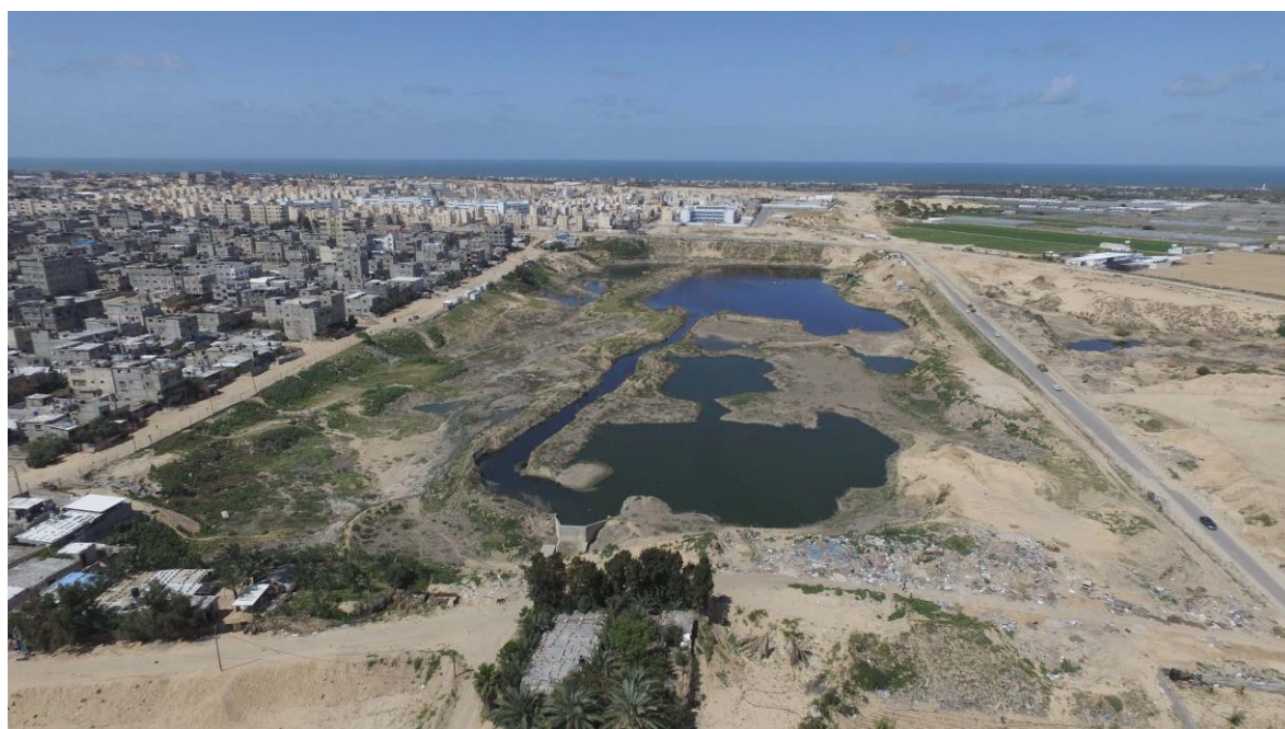
Al Amal Lagoon (Before the intervention)
