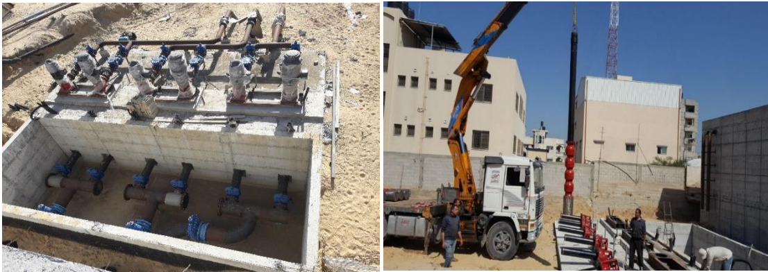
Figure 15: Blending Tank (Al Sheikh Radwan Water Tank)
