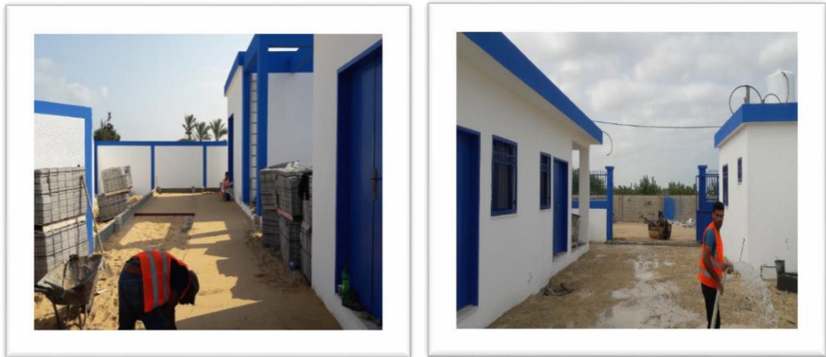
Figure 32: Al Zahra sewage pumping station
