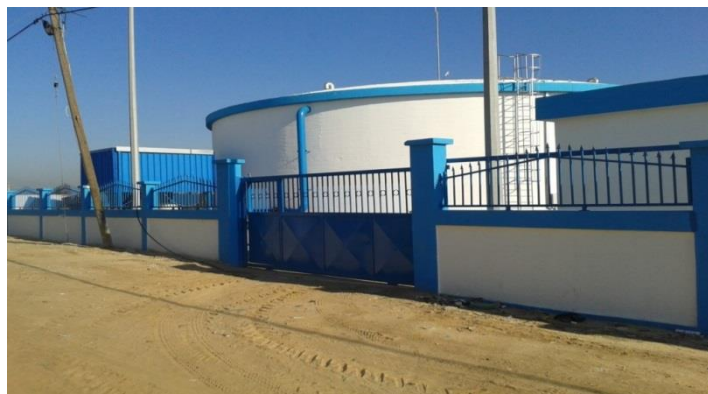
Figure 24: Al Moghraka Water tank
