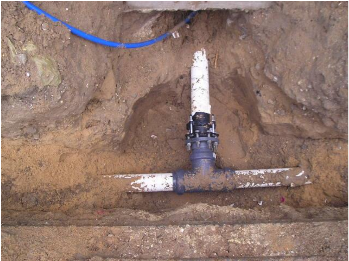
Figure 2 : Water networks Repairs and installations
