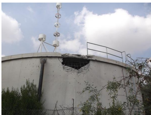
Figure 26: Damaged Water tanks
