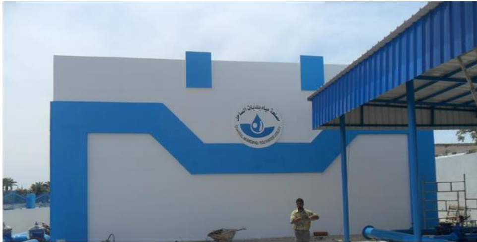
Figure 25: Al Aqsa Water Tank - Dair El Balah
