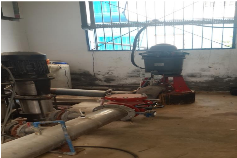
Figure 17 : Construction of and rehabilitation of Bani Suhaila Main Water Booster Station
