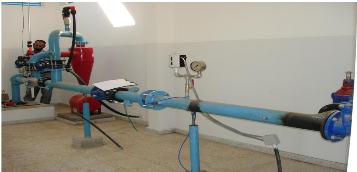
Figure 5 : Drilling and Equipping of a Water Well
