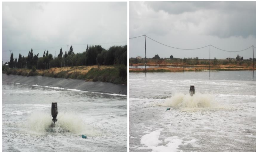
Figure 27: Beit Lahia Wastewater Treatment Plant
