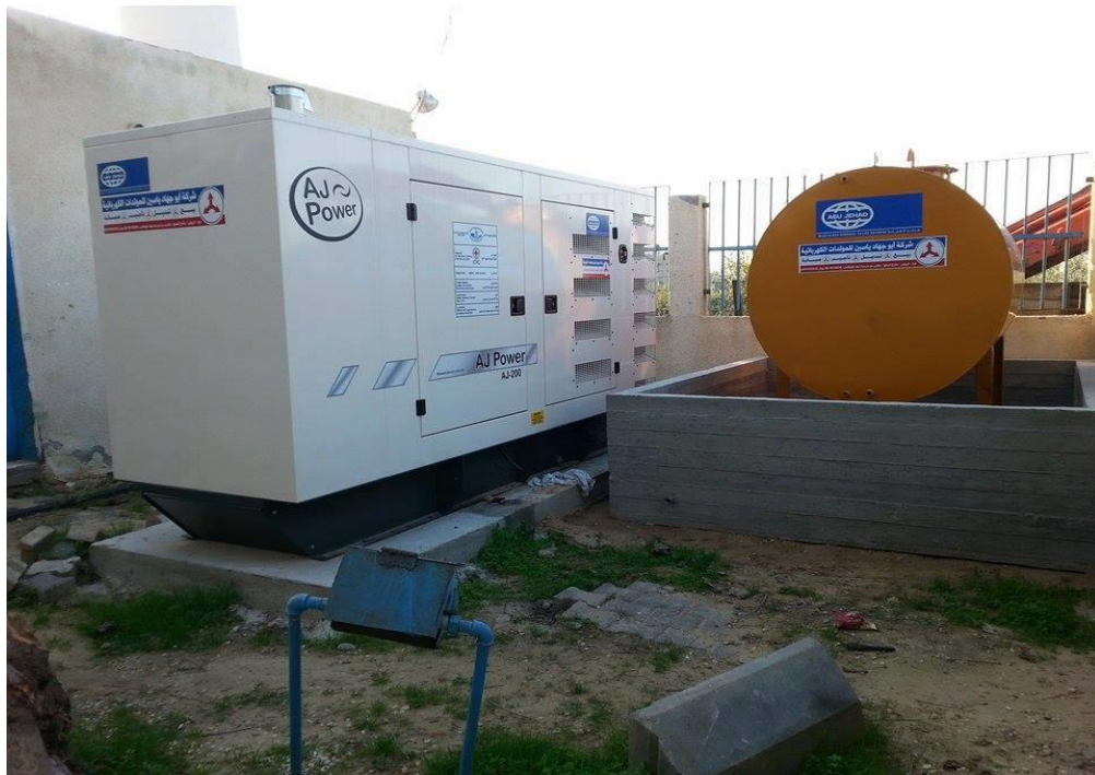
Figure 7: Generator and Fuel Tank Installation in Water Well Facility
