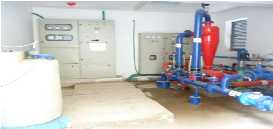
Figure 18: Rehabilitation of Water Well
