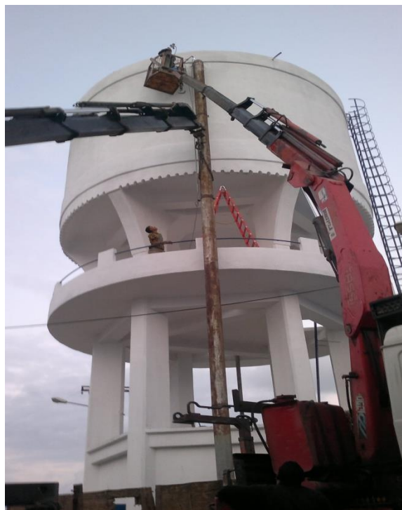
Figure 20: Repair and rehabilitation of elevated tank in Khanyounis -Sadda Desalination site
