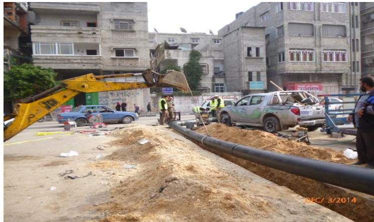
Figure 32: Emergency HDPE Carrier Line – Gaza City
