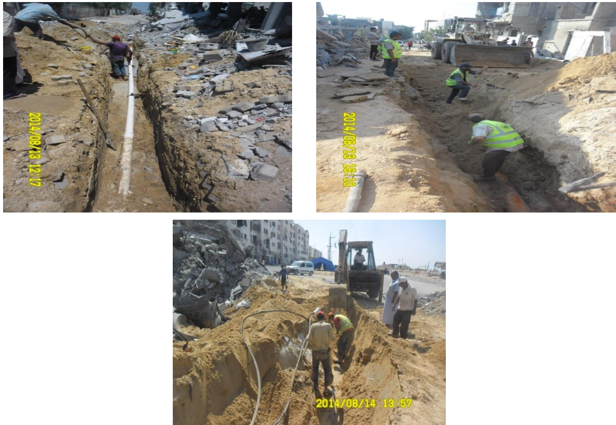
Figure 23: Rehabilitation works After War
