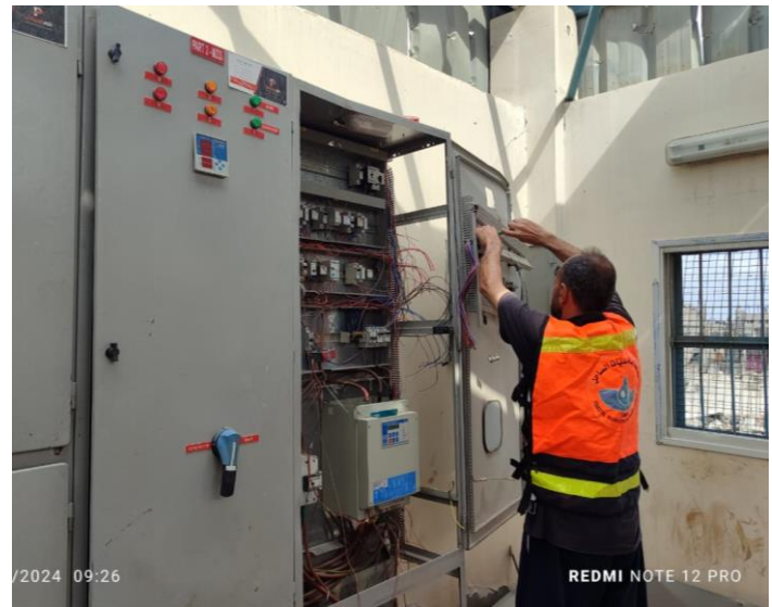
Repairing of the Electrical panels for 4 Water Wells in Khan Younis (Maan, Aya, Hamad 2 and Hamad 3)
