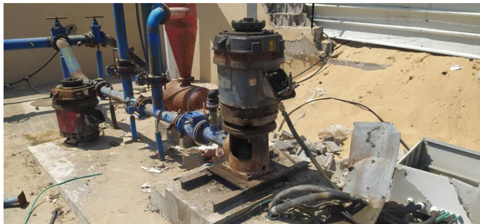
Maintenace and repair works for Al Satar water well 60 m 3 /hr capacity.
