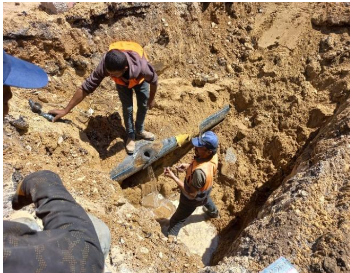
Repairs in Emergencies – Gaza City
