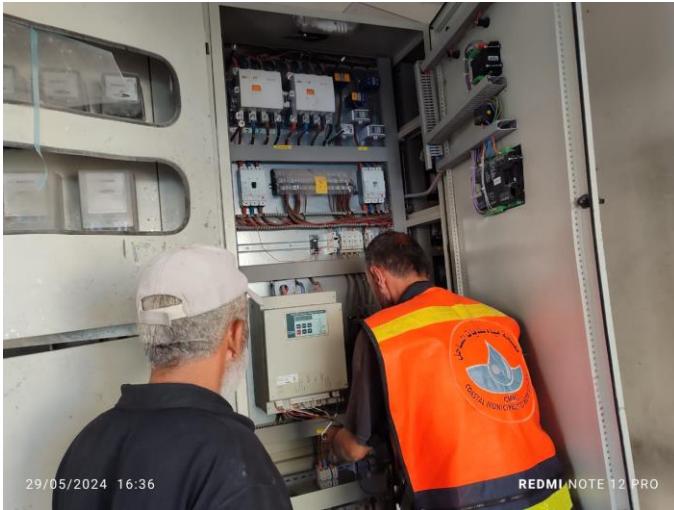
Repairs for damaged panel boards of water and Wastewater Facilities (Al-Saada Desalination Plant, Al-Mazlaqan Well, Al-Saada Well, Al-Israa Tank)
