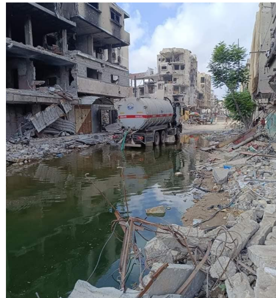
Deplment of CMWU Sewage Vacume trucks to work in Khan Younis and Deir El Balah areas.
