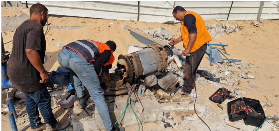
Maintenance works for G-49 water wells in Al Nusairat
