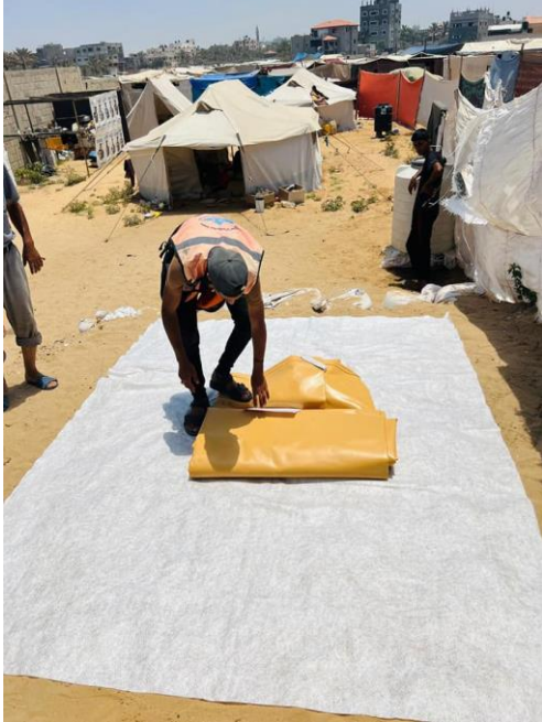
Installation of Water Bladders (Rubber Storage Tanks) in AlQarara, Khn Younis, Abasa, Deir El Balah 5 and 10 cubic eters volume
