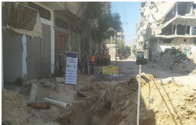
Repair Works at Al Burej
