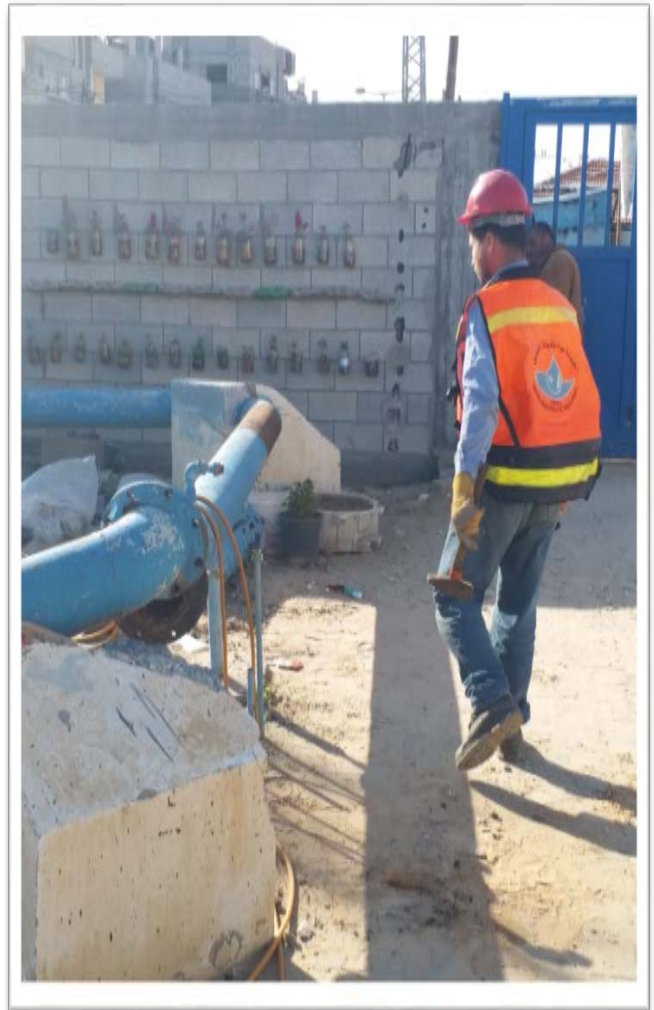
Figure 11 Part of mobile mechanical maintenance and repair workshop activities
