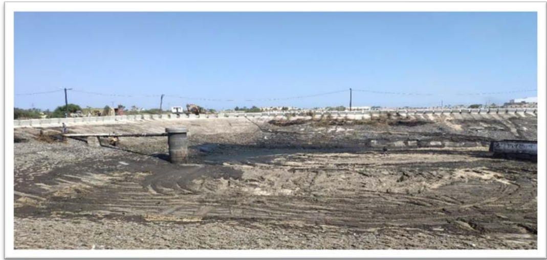
Figure 25 Cleaning of anaerobic wastewater lagoons –Rafah wastewater treatment plant
