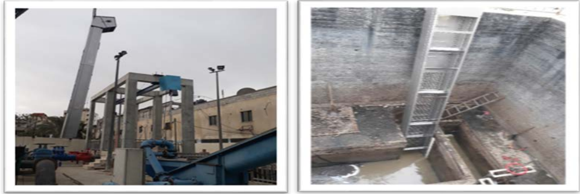
Figure 35 Installing mechanical Bar Screen at Hesbit Alsamak PS
