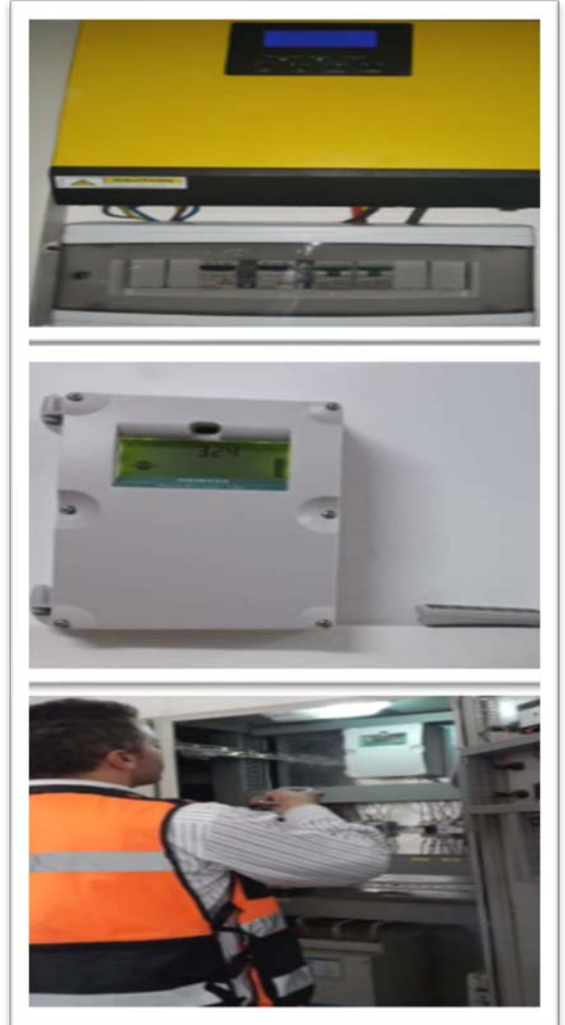
Figure 6 Part of the upgrading activities
