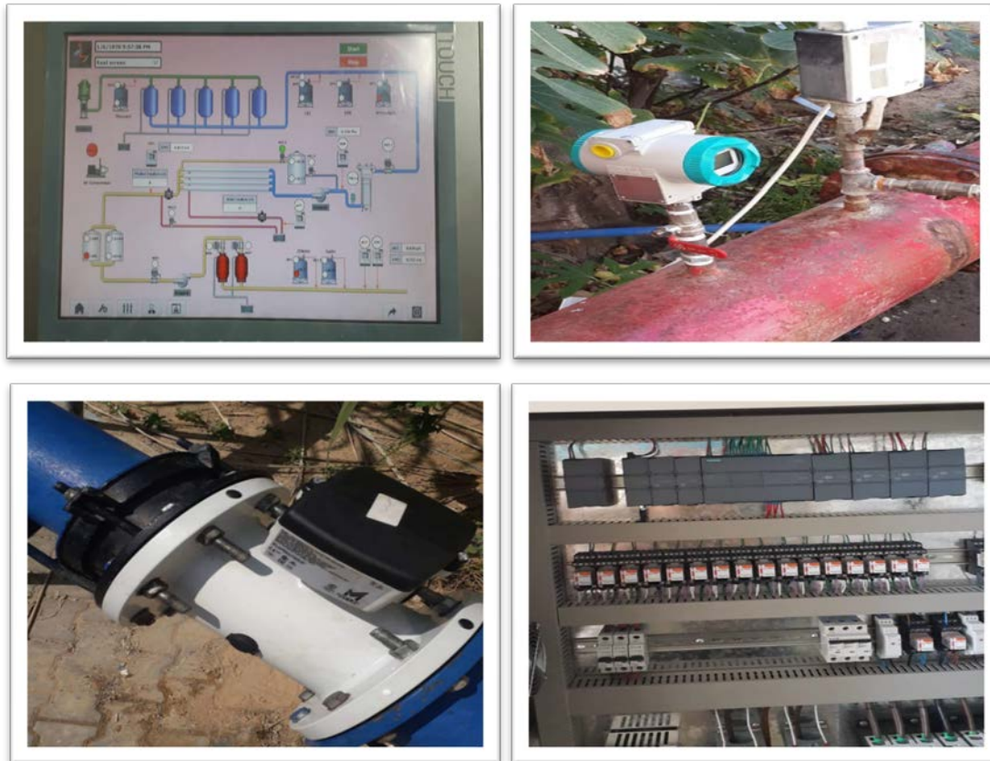
Figure 9 SCADA system for water wells
