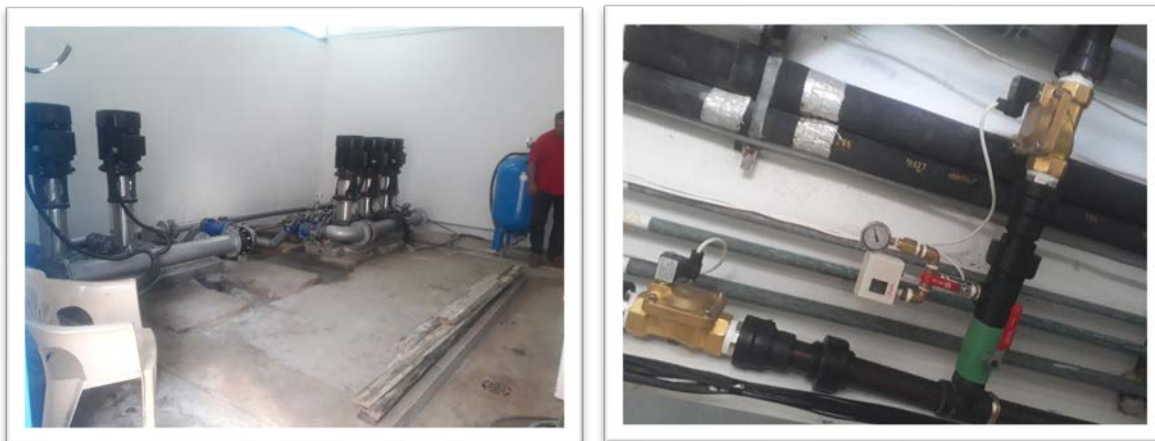
Figure 22 Rehabilitation of Al Shifa water network
