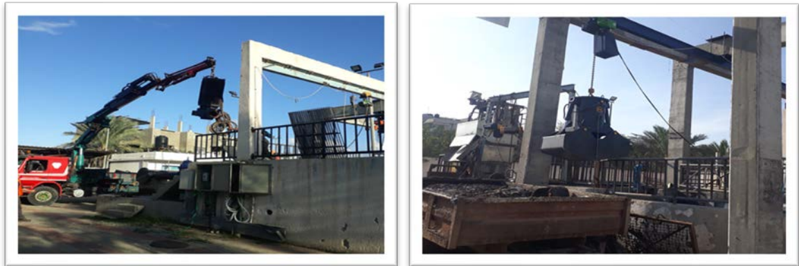
Figure 36 Installing sand removal clam shell at Al Wafia PS
