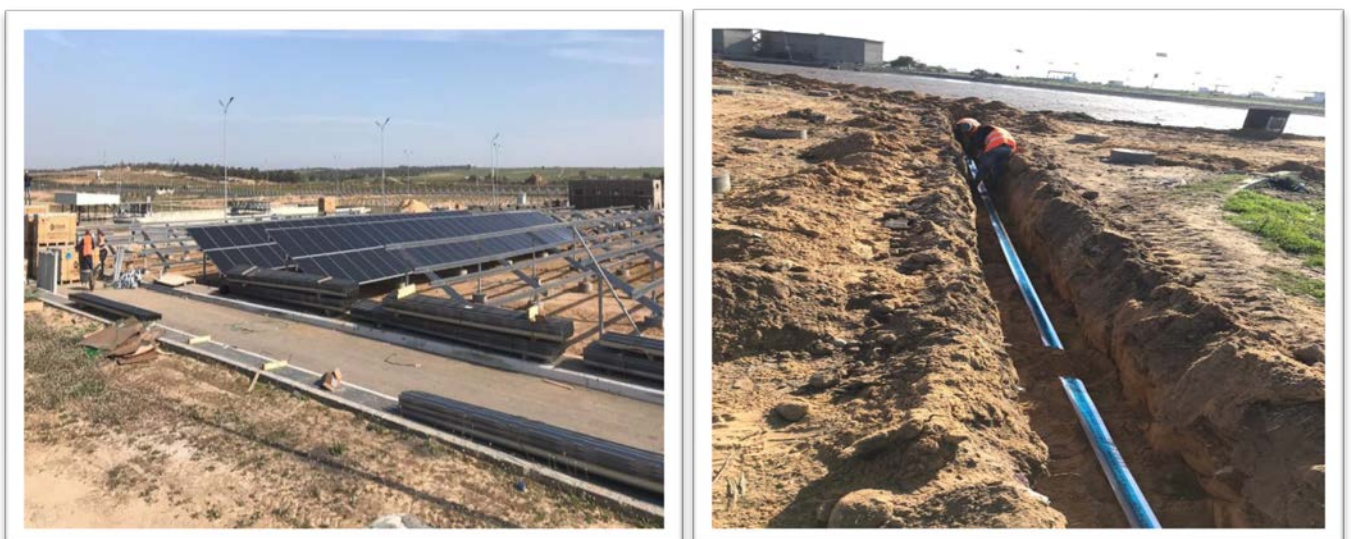
Figure 28 Solar Panels installation
