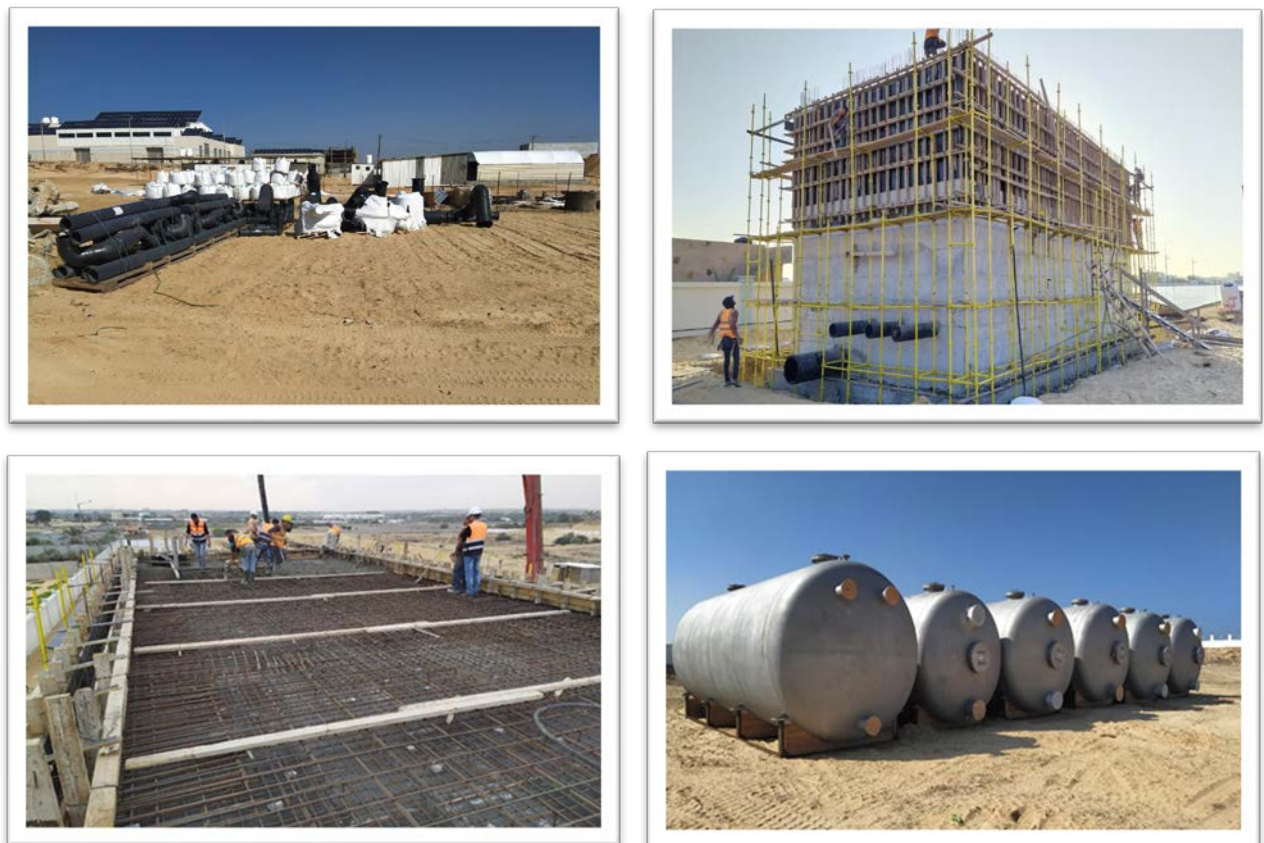
Figure 17 Ongoing activities at Sea Water Desalination Plant – Southern Governorates
