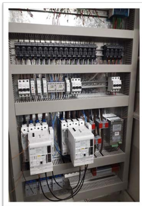
Figure 8 Part of SCADA Works
