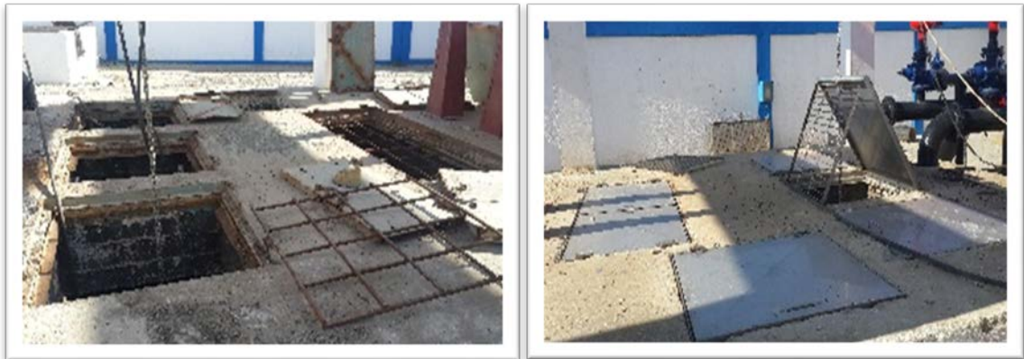
Figure 37 Sewage PS repairs
