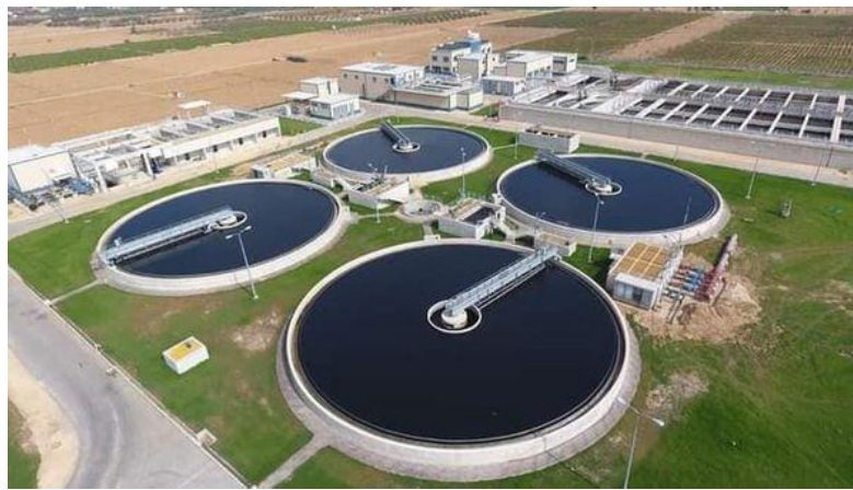
Figure 33 Central WWTP and Central PS Wadi Gaza
