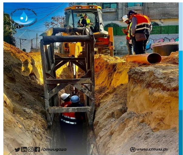
separation between stormwater and WW networks-Jabalia
