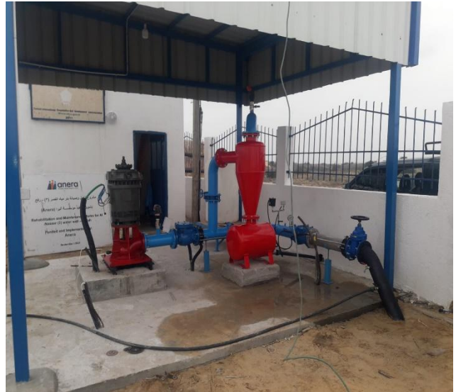
Figure3: Upgrading of Al naser 3 well – Al naser
