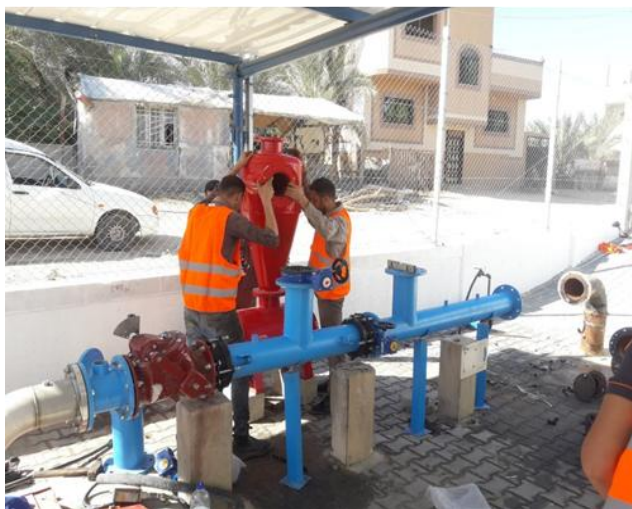
Figure4: Replacement of K-19 well's manifold – Al Qarara
