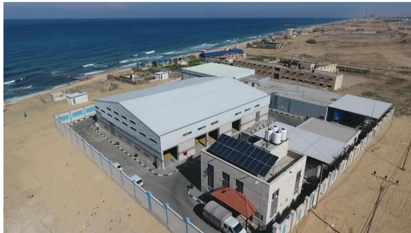
Figure 24 Gaza STL Desalination plant
