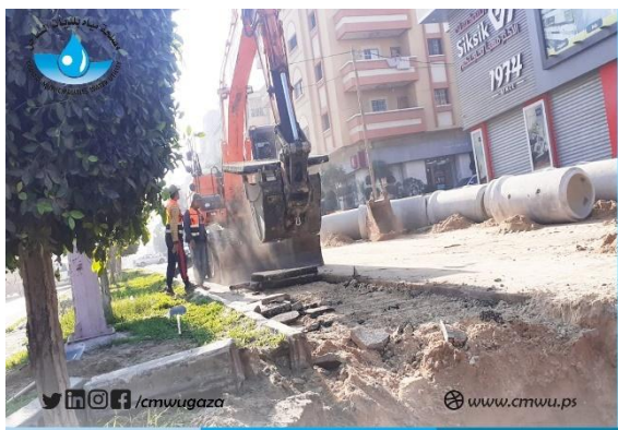
Figur**: Stormwater pipeline from Sheikh Zayed basin to the main collector of Al mashroua basin
