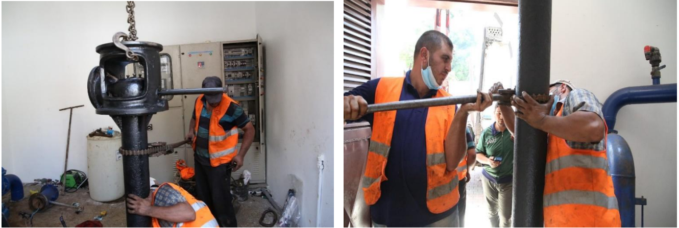
Figure2: Rehabilitation of Omari well - Jabalia
