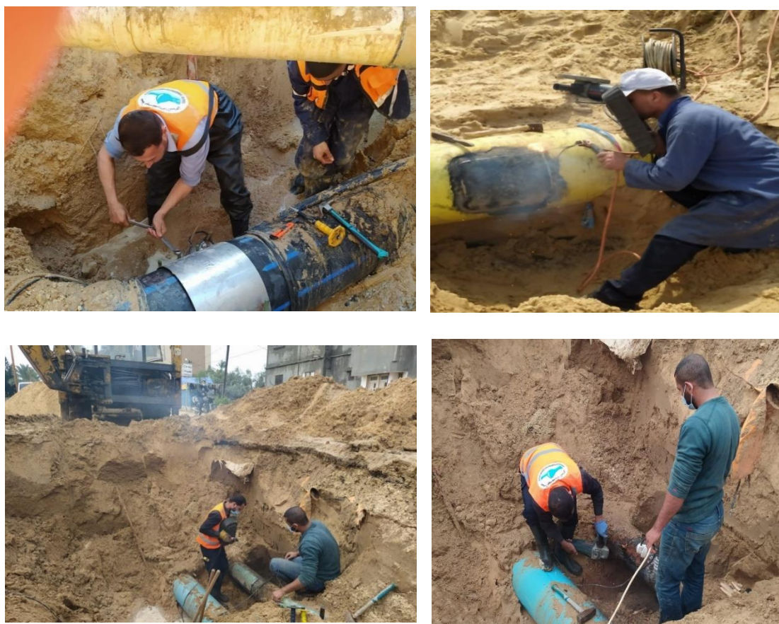
Figure 17 Part of mobile mechanical maintenance and repair workshop activities
