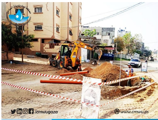
separation between stormwater and WW networks-Jabalia
