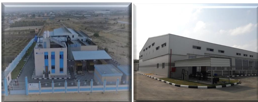
Figure 22 Sea Water Desalination Plant – Southern Governorates
