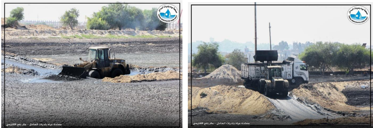
Figure 32 Cleaning of anaerobic wastewater lagoons –Rafah wastewater treatment plant
