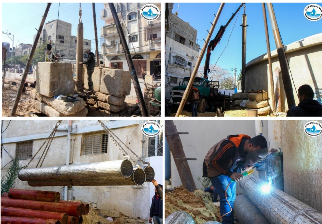
Figure7: Construction Water Wells at Rafah
