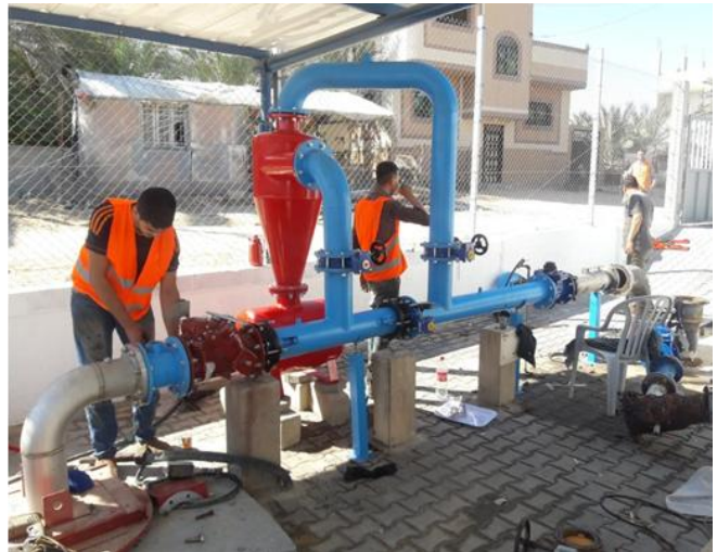
Figure4: Replacement of K-19 well's manifold – Al Qarara
