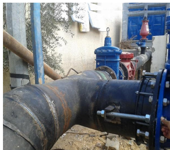
Figure 35: HDPE pipeline from Jomizit Al Sabeel PS to WWTP at Rafah
