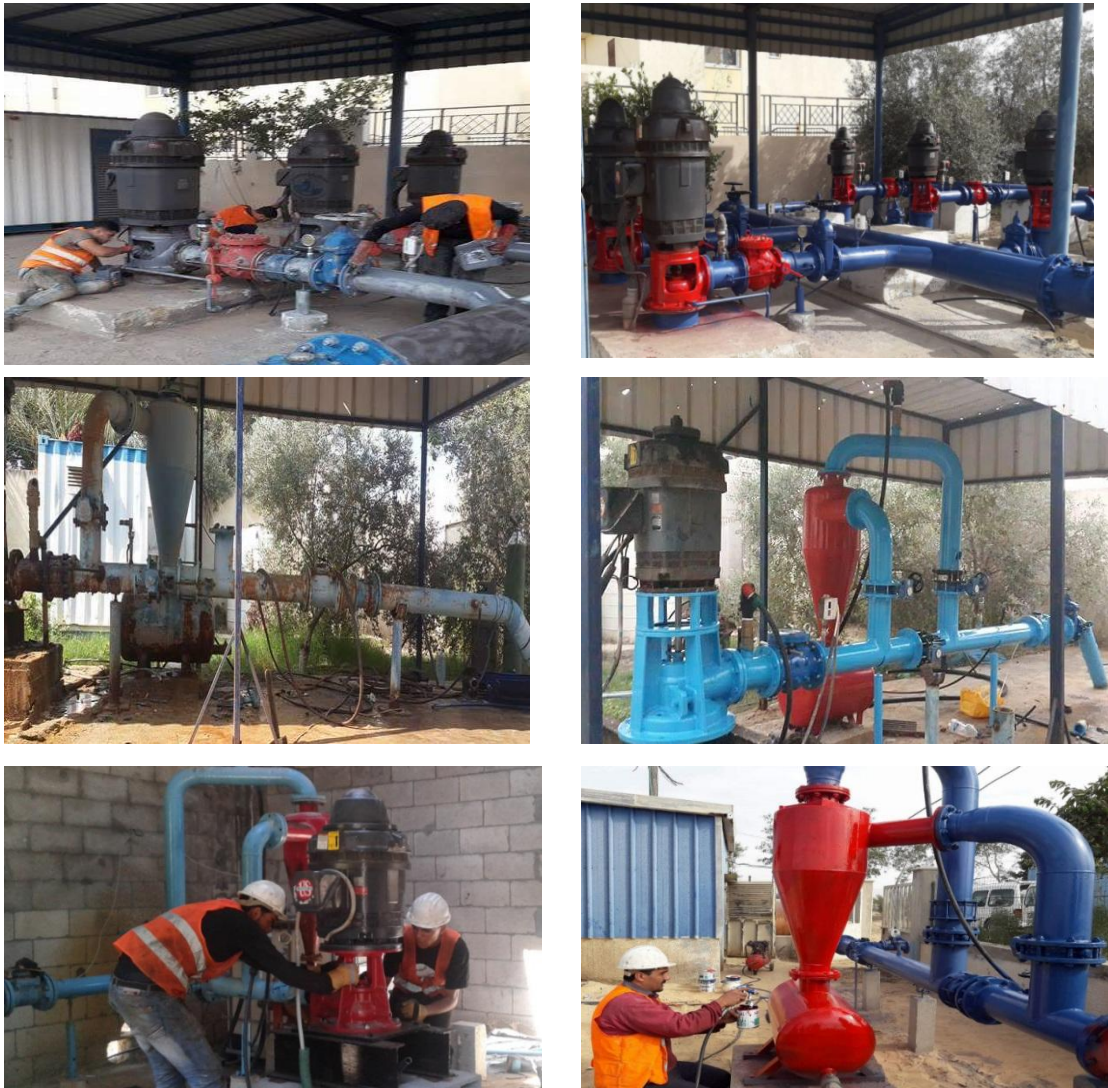
Figure 8: Water facilities Repair, Refurbishment and Rehabilitation Works
