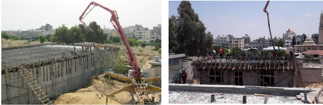
Figure 17: Blending Tank (Al Sheikh Radwan Water Tank)
