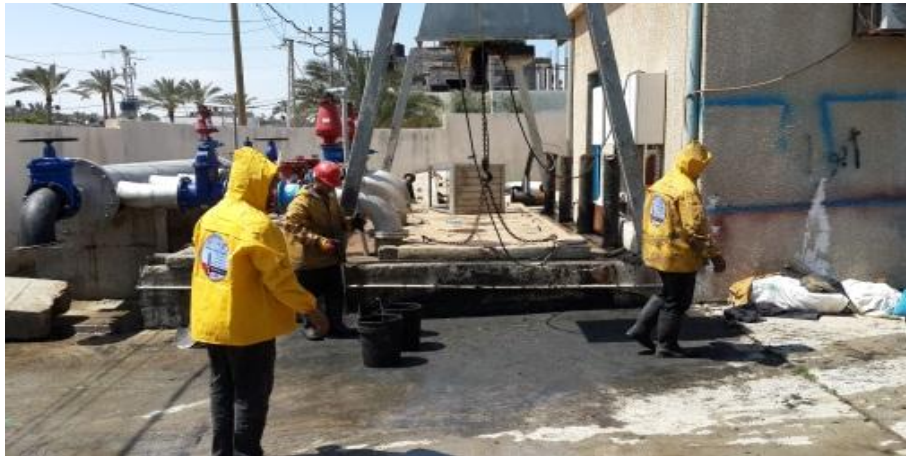
Figure 43 : Cleaning Pumping Station Yard
