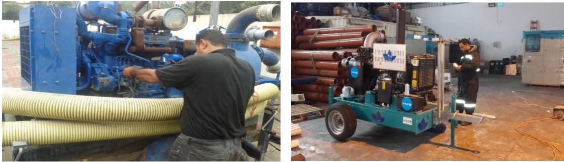
Figure 44: Mobile Pumps Maintenance
