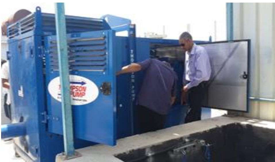
Figure 47: Repair Enjaily Strom Water P S Generator
