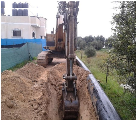
Figure 35: HDPE pipeline from Jomizit Al Sabeel PS to WWTP at Rafah
