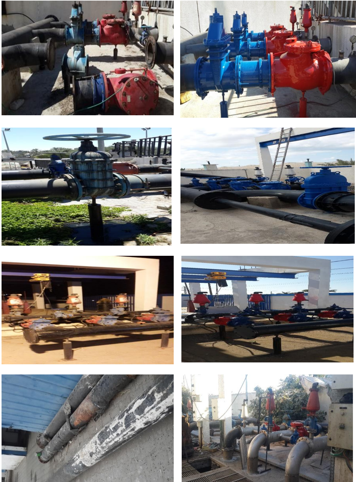
Figure 40: Maintenance of Pump's Manifolds
