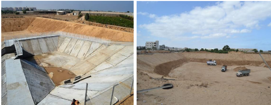
Al Qarar Figure 32: Al Qarara Storm Water Project
