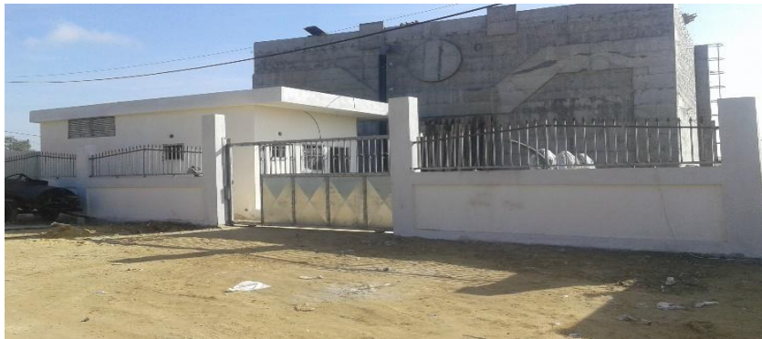
Figure 24: Abasan Water tank
