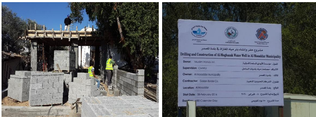
Figure 6: Al Mosadar water well
