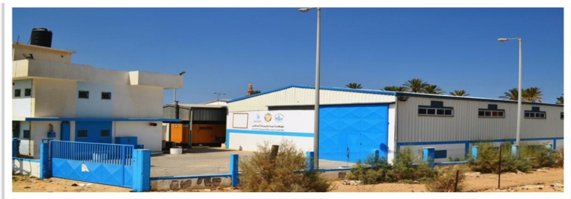
Figure 15: Deir Al Balah Sea Water Desalination Plant
