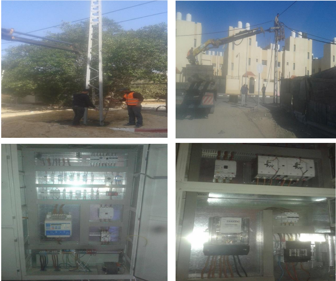
Figure 7: Part of Electrical works
