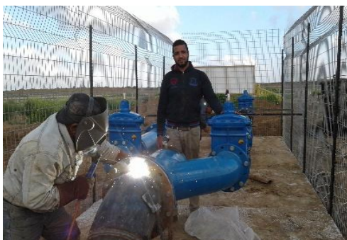
Figure2: Water networks Repairs and installations
