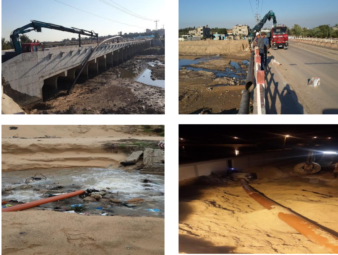
Figure 41: Emergency Repairs for Wastewater Pressure Lines
