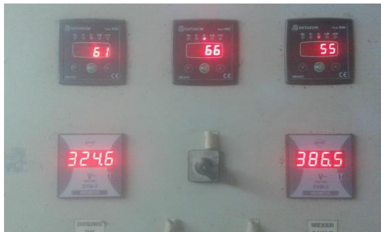
Figure 12: Well head Electric Stabilizer-Voltage Step up Transformer connections
