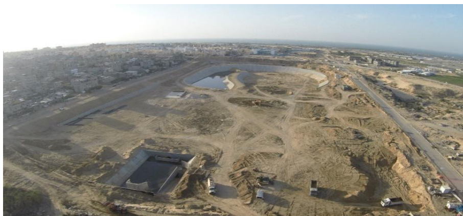
Figure 29: Al Amal Storm Water Project
