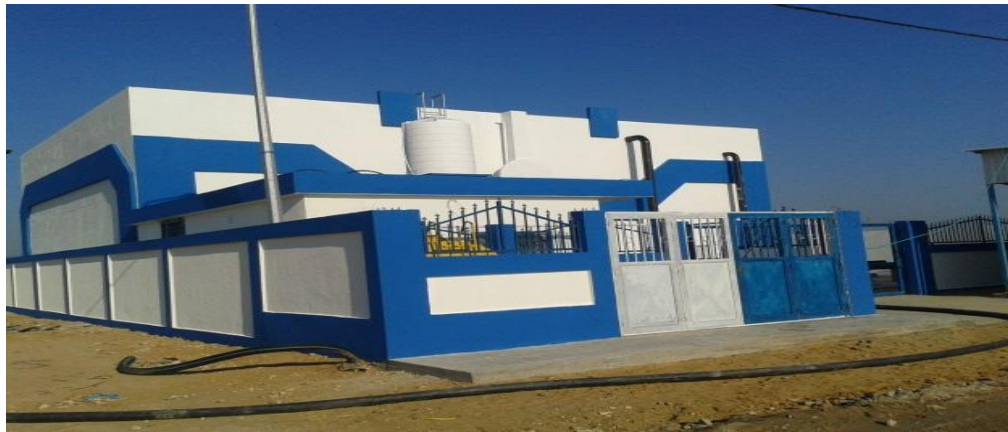
Figure 22: Khuzaa Re-constructed Water Tank
