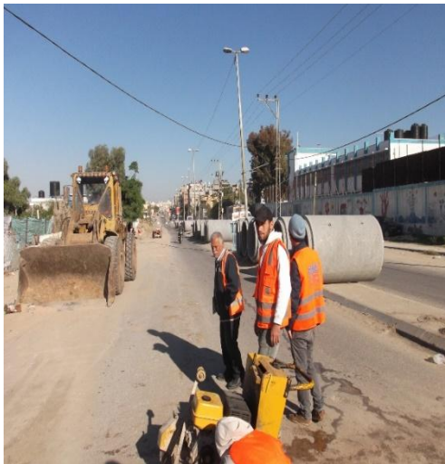
Figure 31:Construction Storm water Carrier line-Rafah
