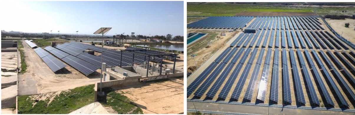
Figure 36 Solar Panels installation
