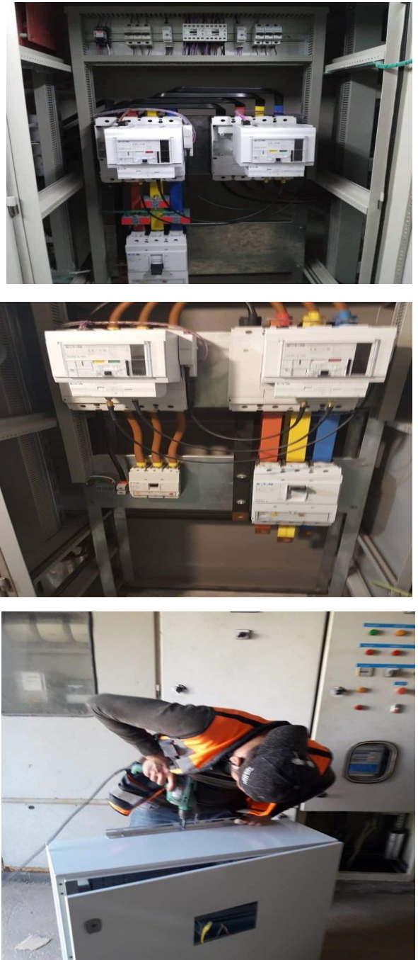
Figure 8: electrical upgrading works
