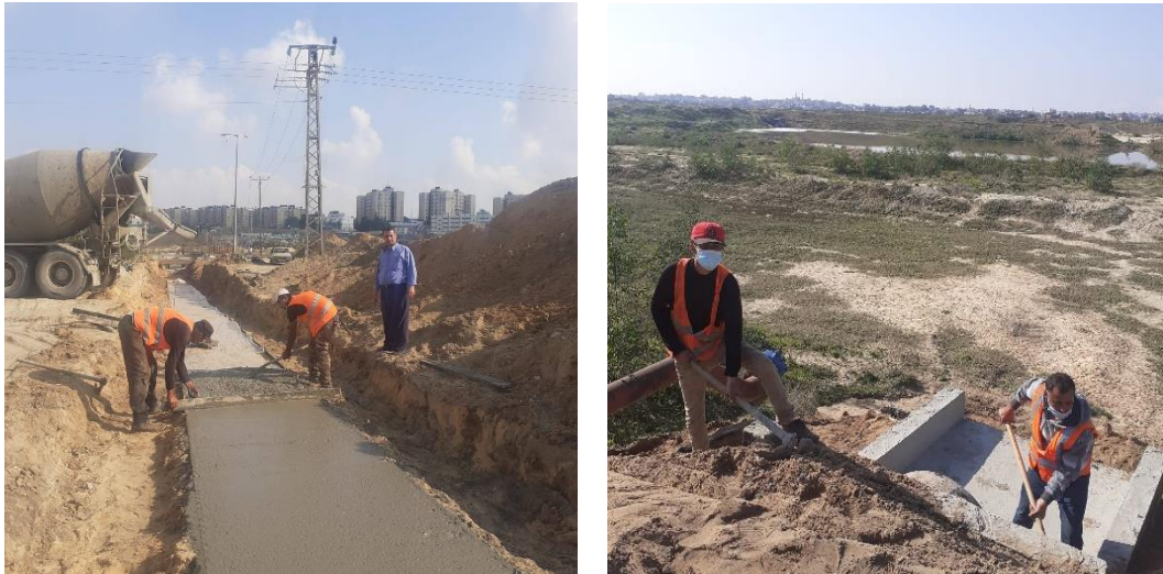
Figure 30 BLWWTP terminal pumping station Spare parts and maintenance activities
