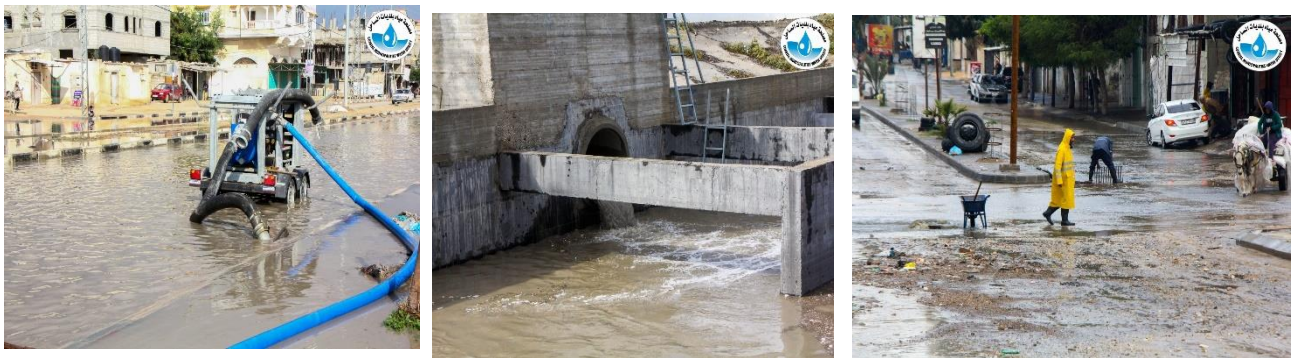
Figure 45 Storm water preparedness activities
