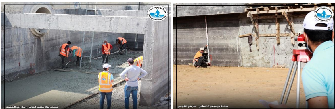
Figure 42 Upgrading works in Al Juninah stormwater basin-Rafah through NRC project
