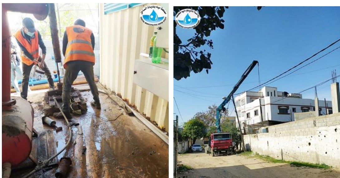
Figure13: Rehabilitation of Al Sabra water well-Gaza city
