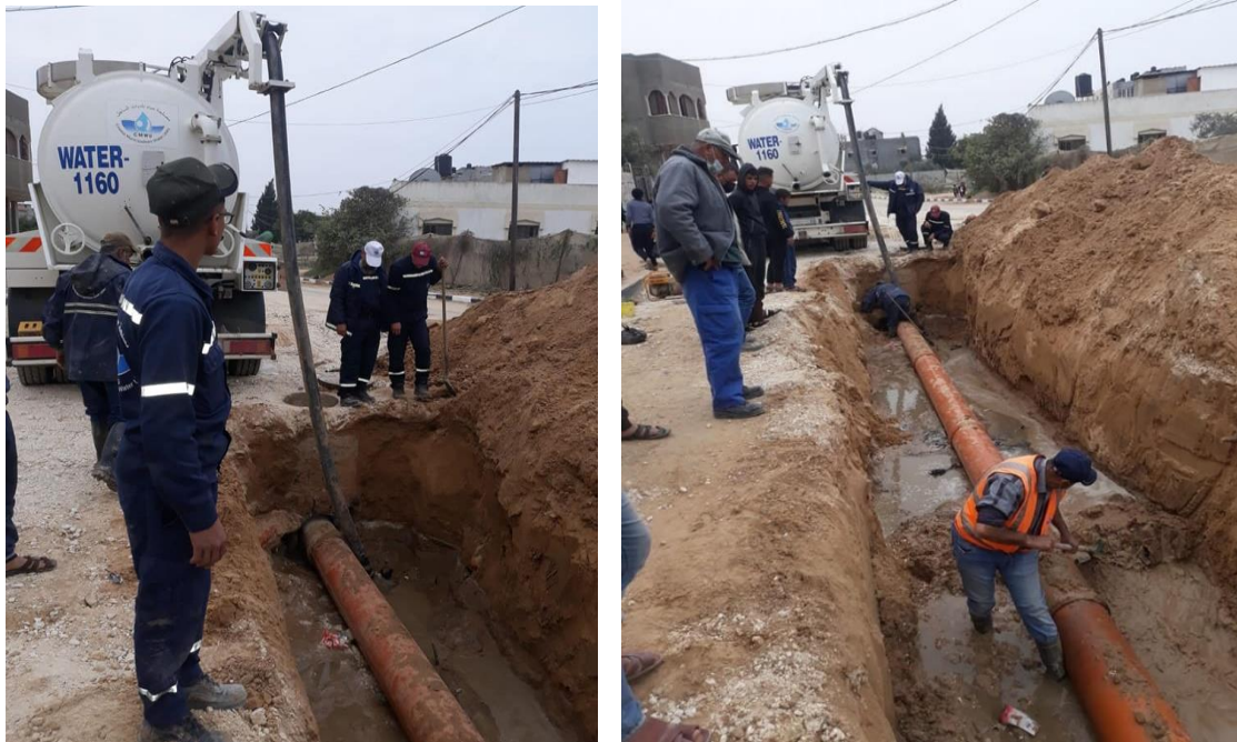
Figure 48 Fixing the damages in wastewater network-Rafah
