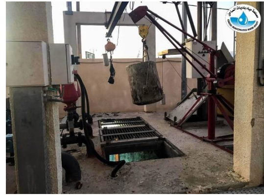
Figure 51: cleaning the pumps room in different sewage pumping stations
