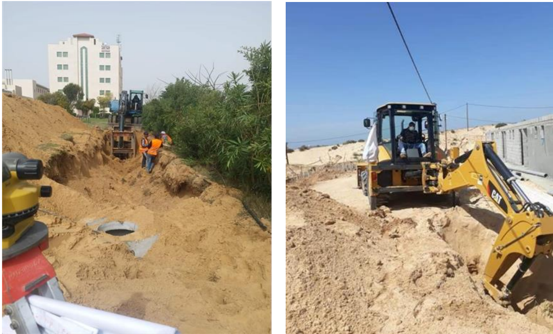
Figure 57 Providing the Quarantine centers with water & WW services
