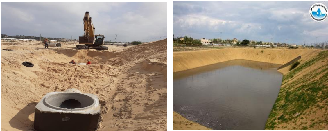
Figure 41: construction of Al Attatra stormwater pipeline and infiltration basin through NRC preparedness project
