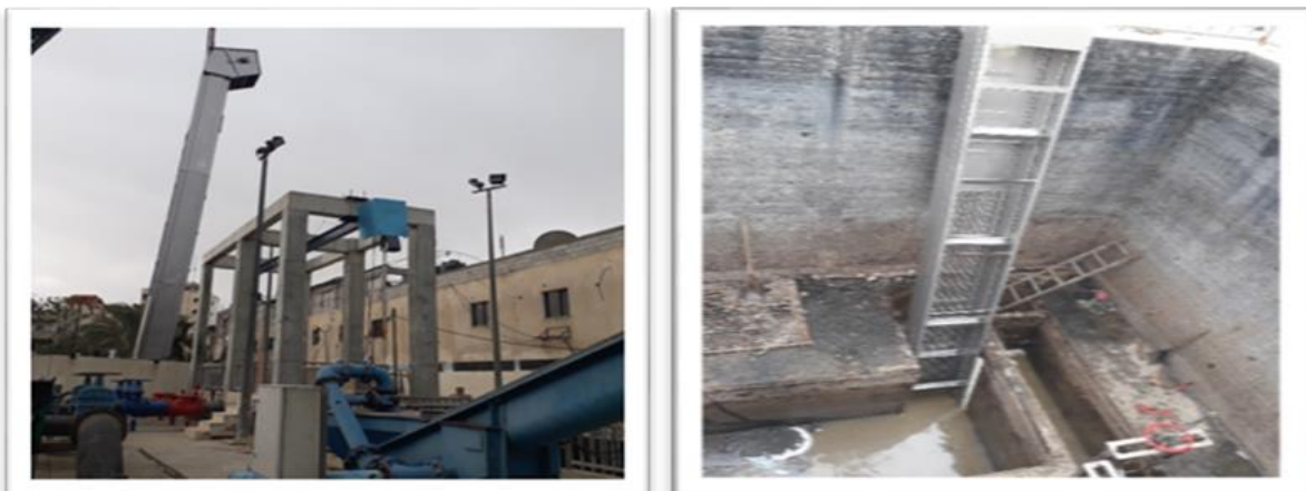
Figure 49 Installing mechanical Bar Screen
