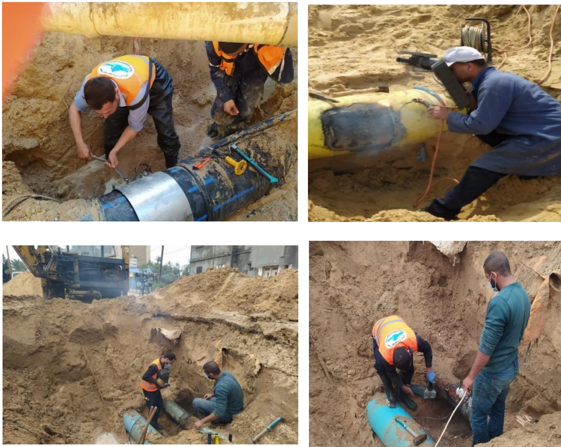
Figure 17 Part of mobile mechanical maintenance and repair workshop activities
