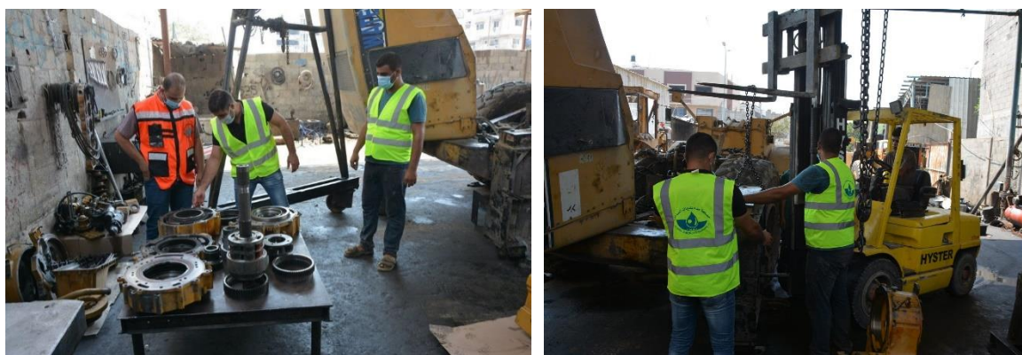
Figure53: Maintenance works for heavy machineries
