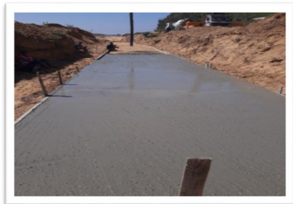
Figure 34 Central WWTP Pressure line
