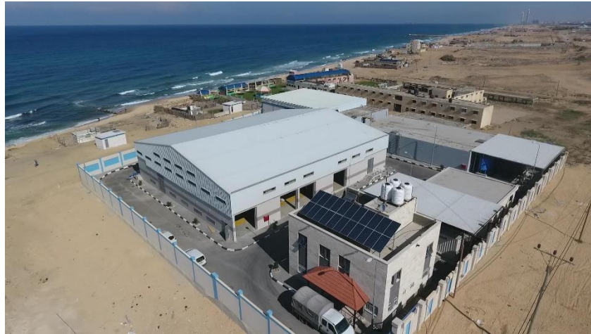
Figure 24 Gaza STL Desalination plant
