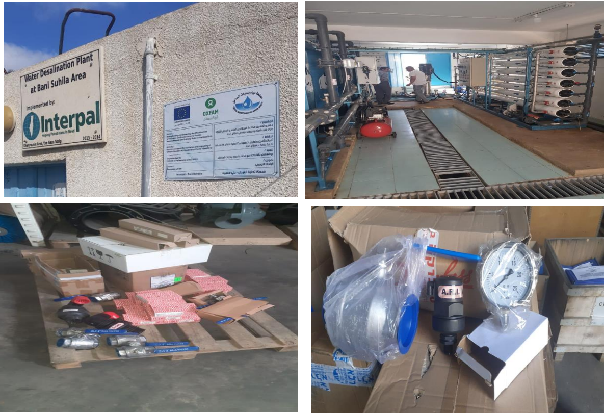
Figure 26 Rehabilitation of brackish RO plants and supply spare parts for RO plants
