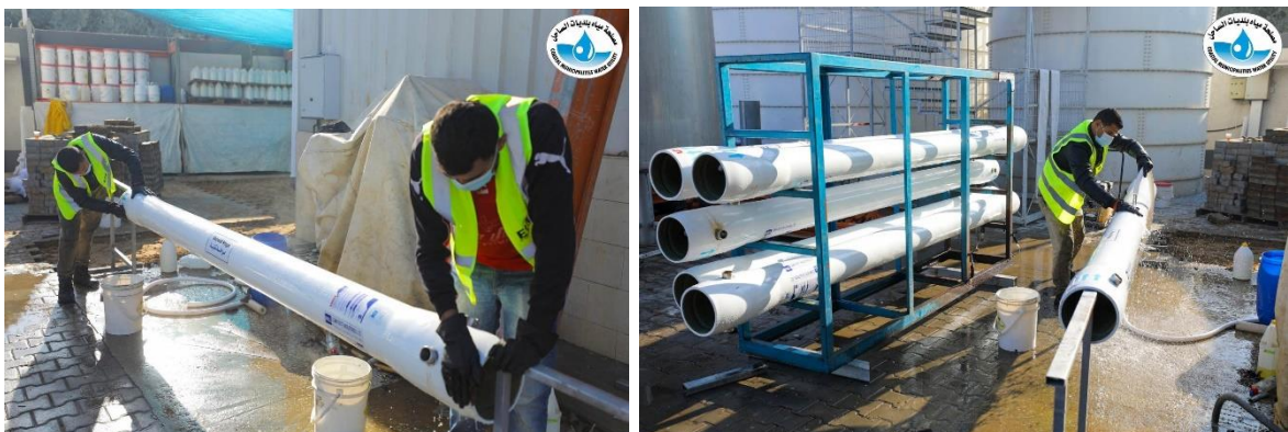
Figure25: rehabilitation of RO plants
