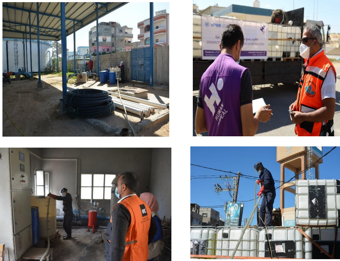
Figure 21 Chlorine solution supply to water facilities
