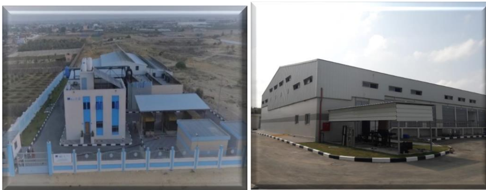
Figure 22 Sea Water Desalination Plant – Southern Governorates
