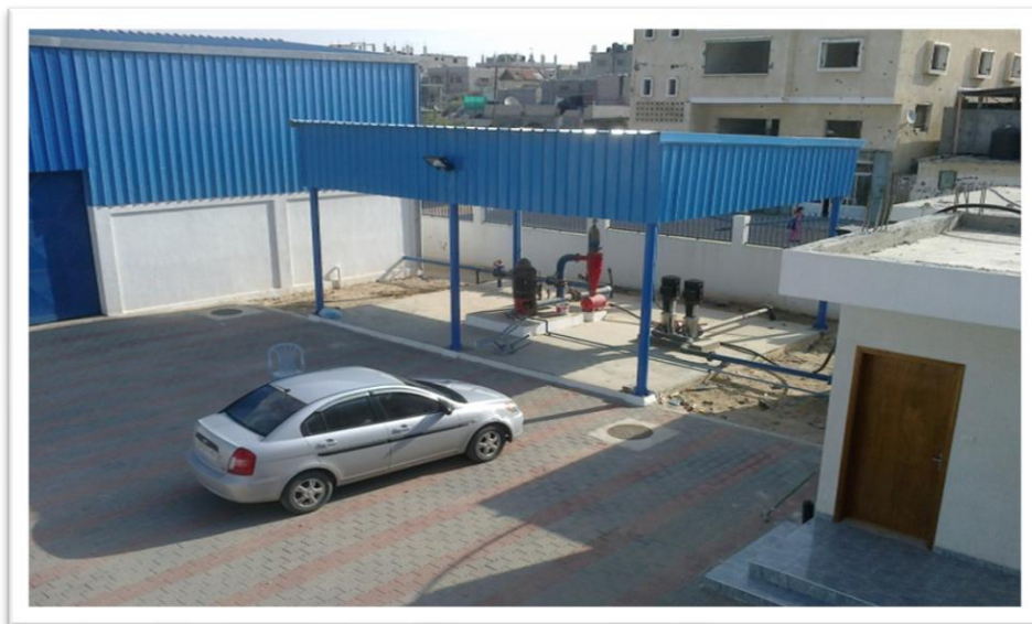
Fig (8) Al Salam Brackish Water Desalination Plant - Rafah
