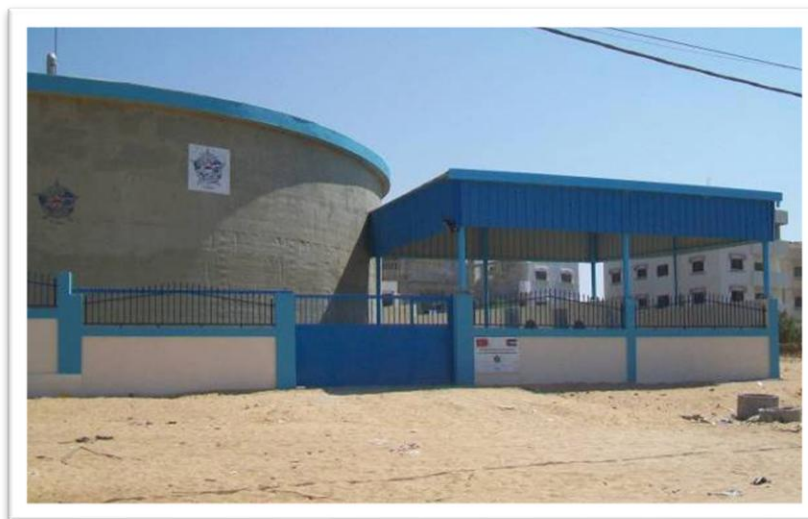
Fig (13) - Water Reservoir in Jabalia
