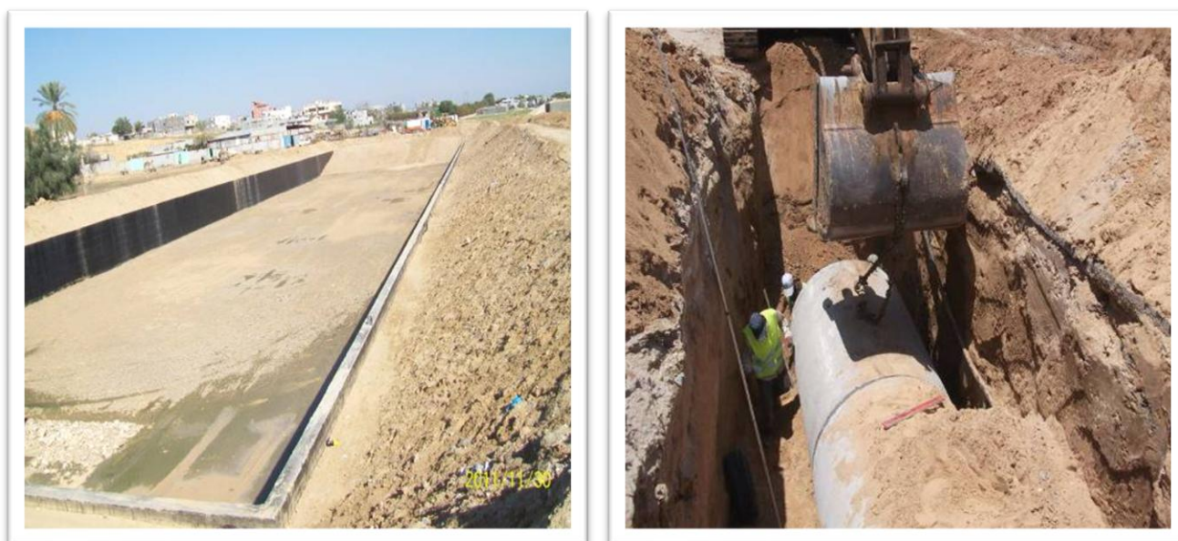
Fig (16) - Construction of Storm water pond and storm water networks at Rafah Area
