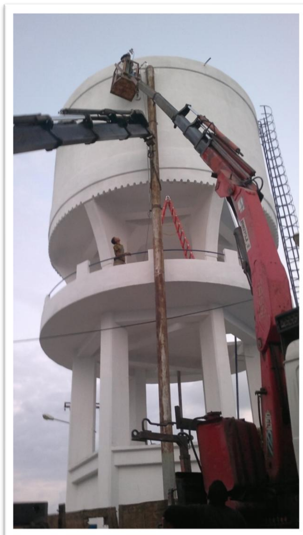
Fig (9) - Rehabilitation of elevated water tank in Khanyounis – Saada Desal. Plant
