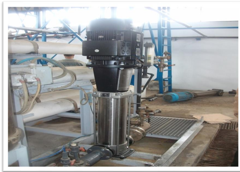
Fig (11) - Repair of high pressure pump- Khanyounis RO desalination plant
