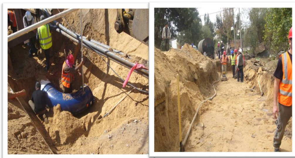
Fig (18) – Construction of Al Hawaber Sewage P.L
