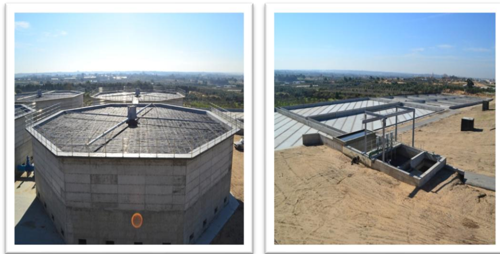
Fig (14) - Gaza Wastewater Treatment Plant
