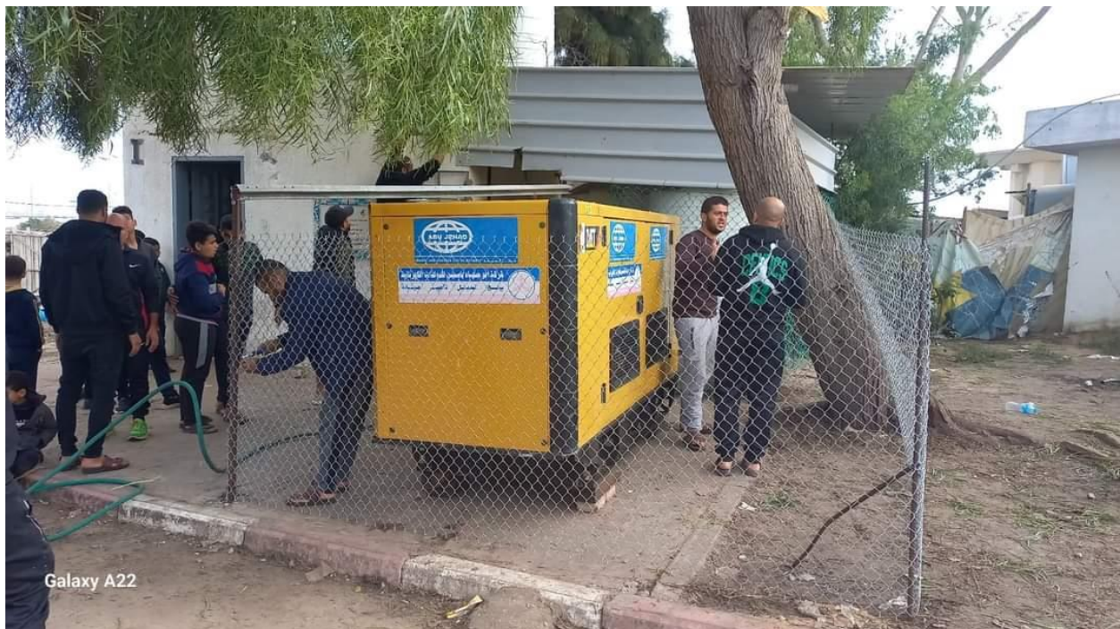
Installation of generator for Al Aqsa university
