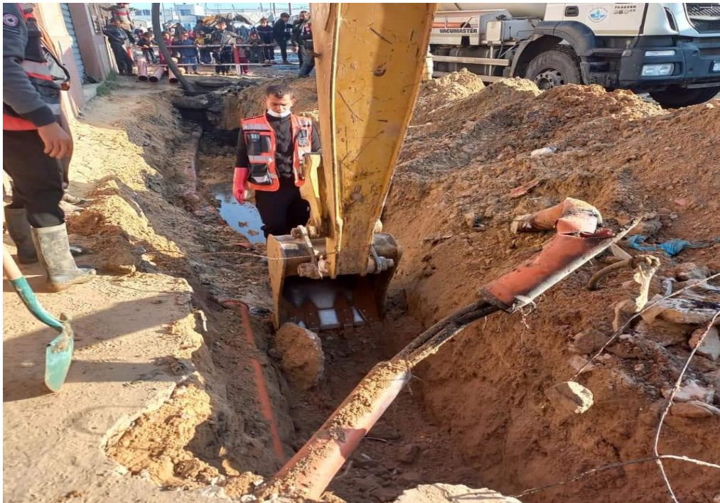
Repairing WW network at Rafah
