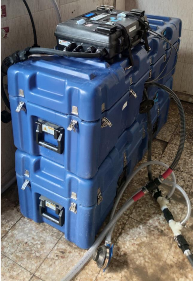
Installation of Desalination units of 16 Cubic Meters /Day
