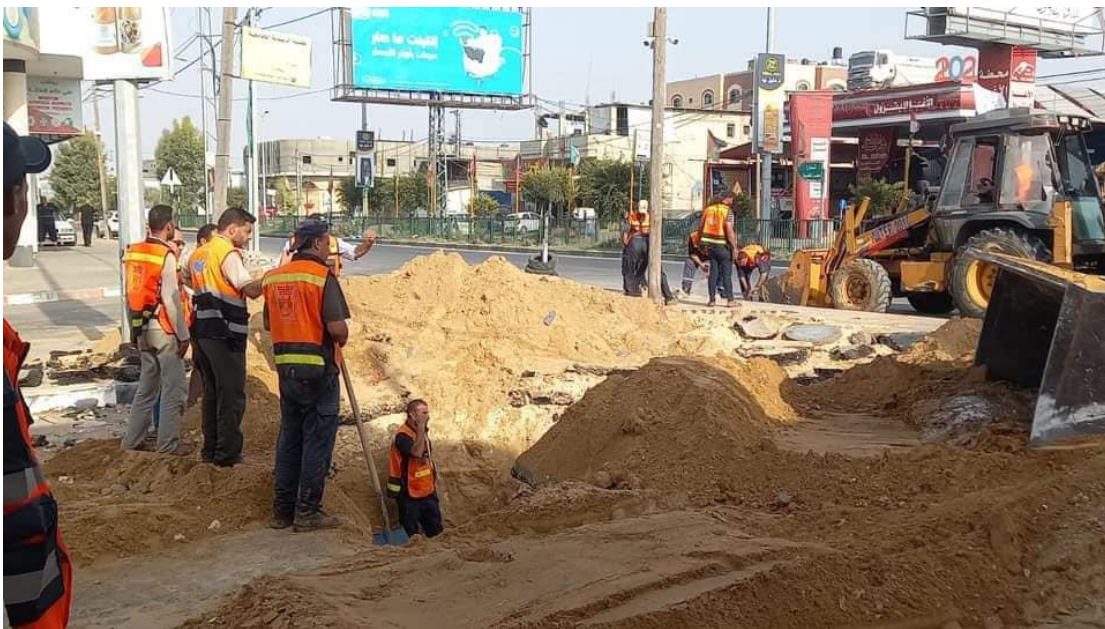
Reparing Water and WW networks at different Areas in Gaza Strip
