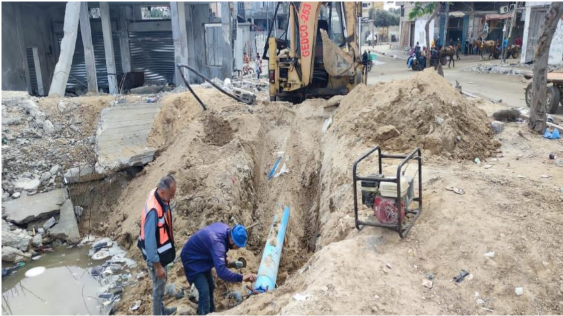
Repairing Mekerot water pipes at Al Nussirat
