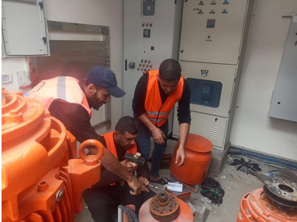
Replacing Water pump-Nusirat
