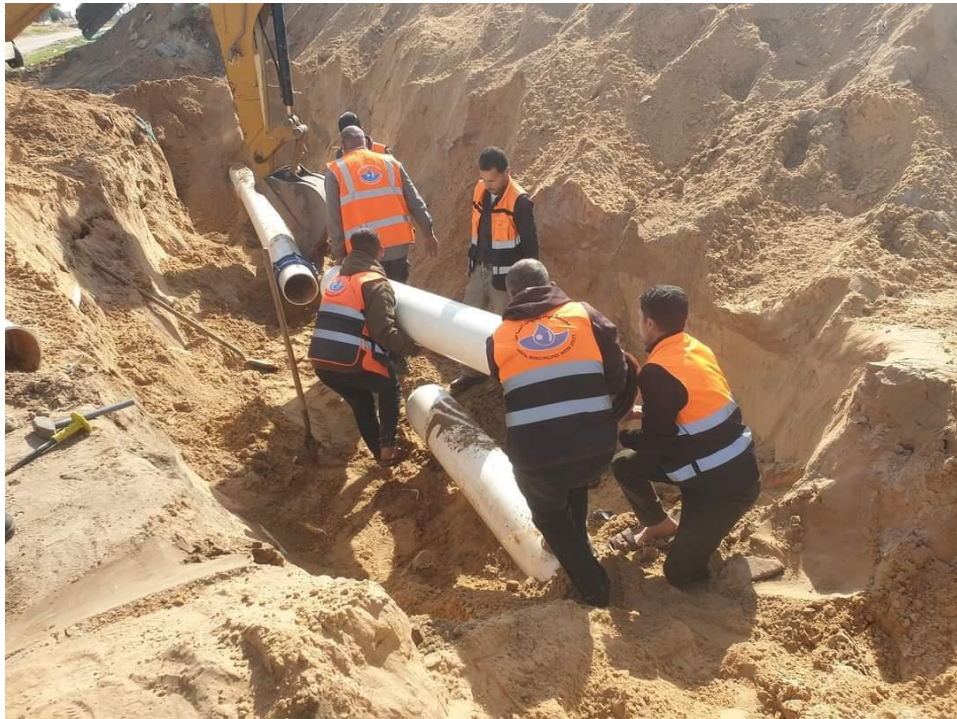
Connecting Mekerot Water pipes to Dair Al Balah
