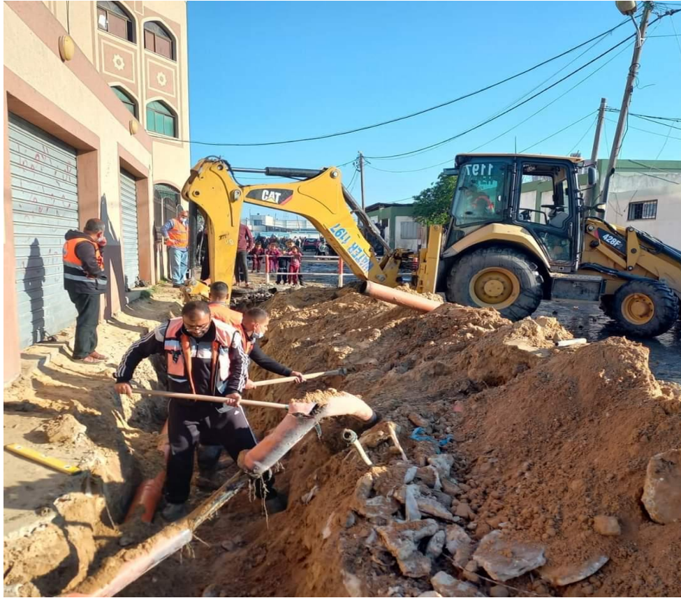
Repairing WW network at Rafah
