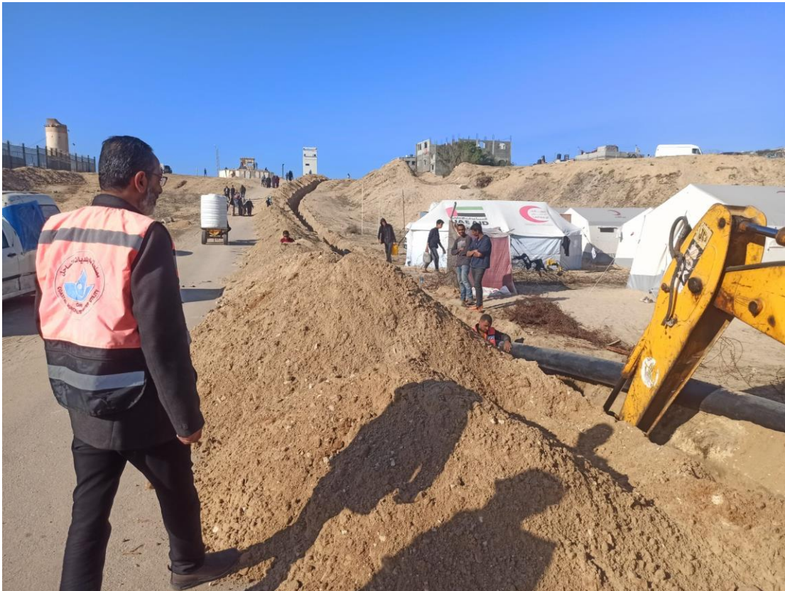
Connecting EUA desalination plant with Water tanks in Rafah area
