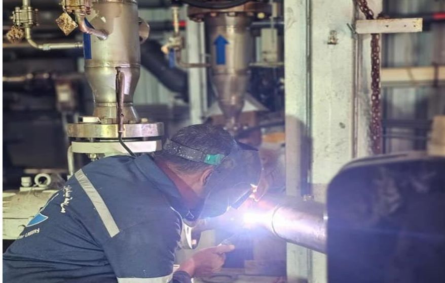
Repairing Al Bassa Seawater Desalination plant-Middle Governorate
