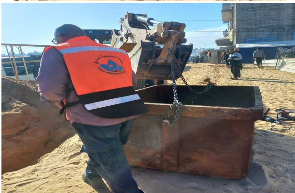
Instalaltion of tepmprary Bathrooms at Rafah
