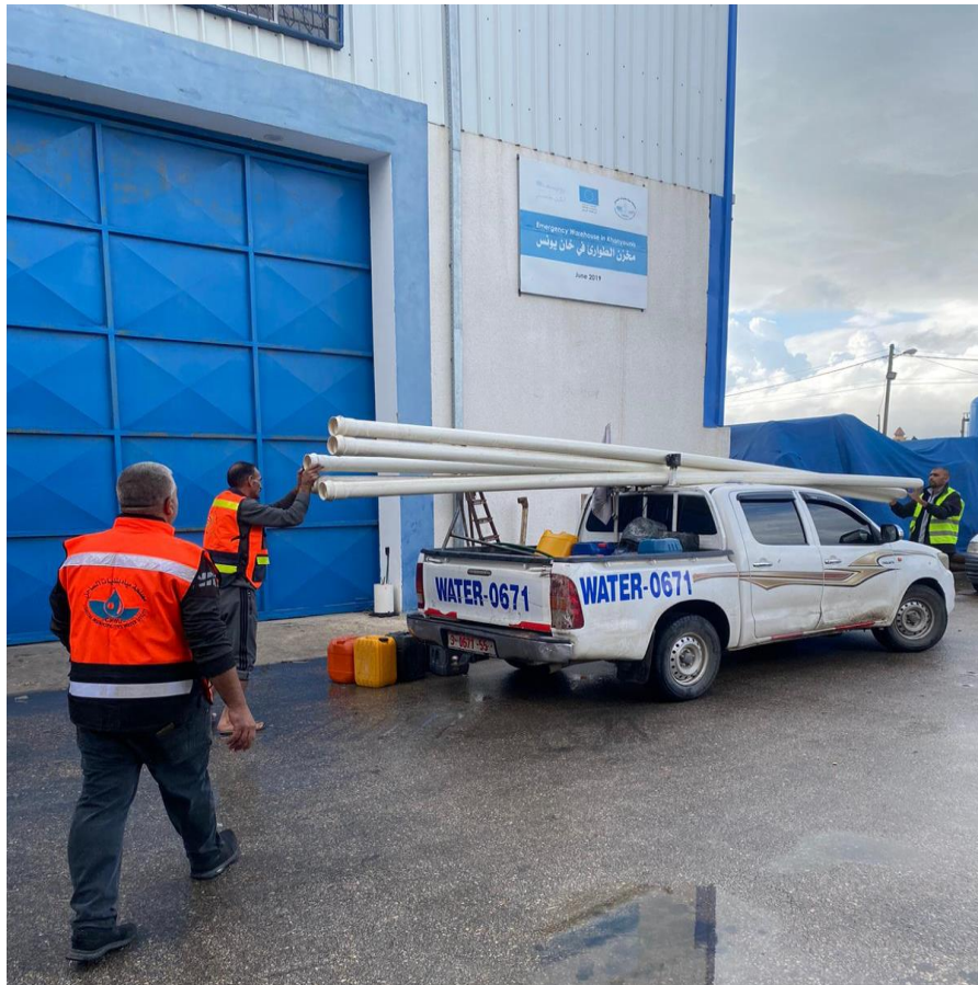
Repairing water networks at Abasan Al Kabera
