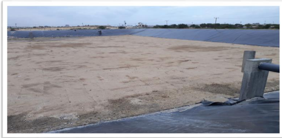
Figure 23: KH Temporary Wastewater Treatment Plant
