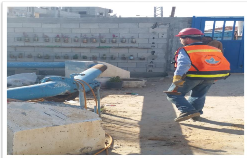
Figure 10: Part of mobile mechanical maintenance and repair workshop activities
