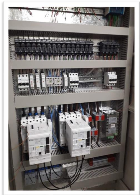
Figure 7:Part of SCADA Works
