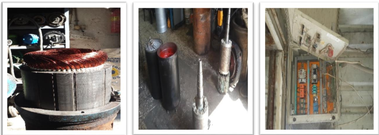
Figure 33: Wastewater electromechanical maintenance
