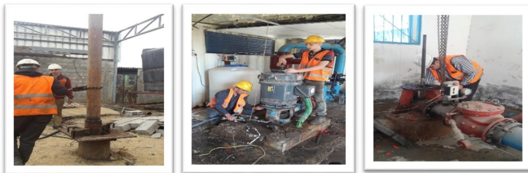
Figure 9: Water facilities Repair, Refurbishment and Rehabilitation Works
