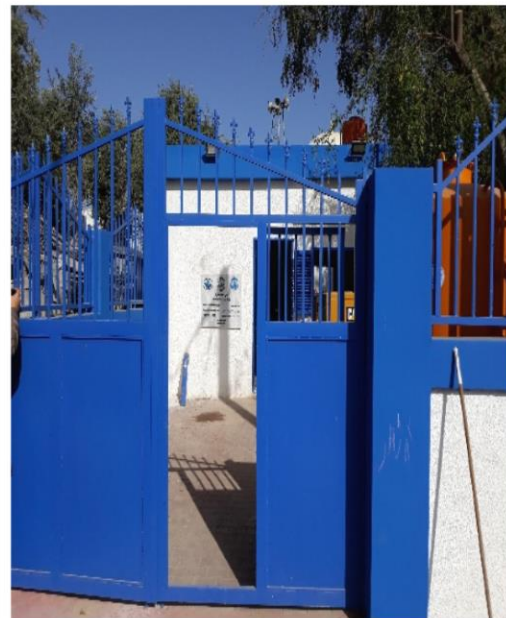
Figure 6: Al Mosader water well
