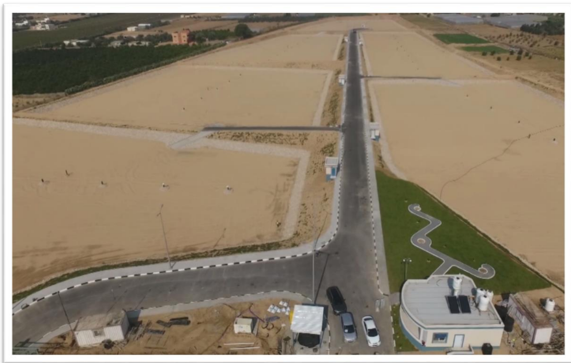
Figure 30: Infiltration Basin at Al Fokhari
