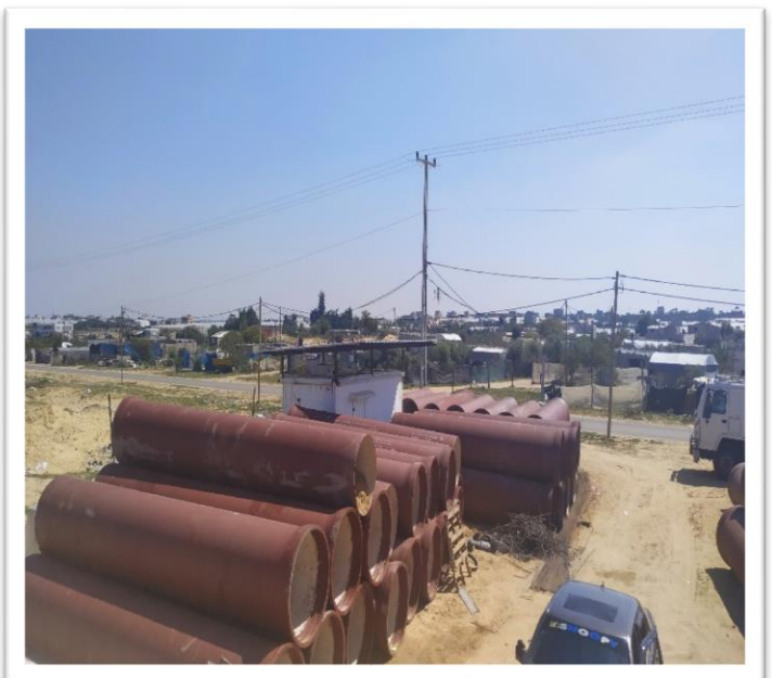
Figure 29: Ductile Iron Pipeline
