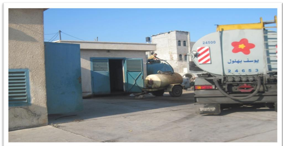
Figure- 14 Fuel Supply and Distribution
