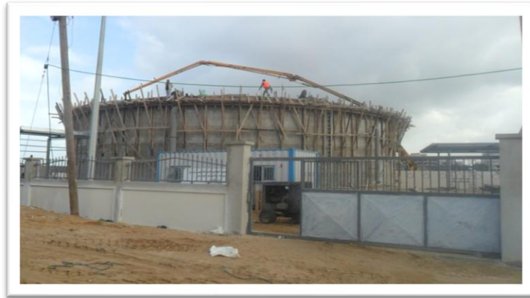
Figure. 18 Construction of Al-Moghraka Water Tank
