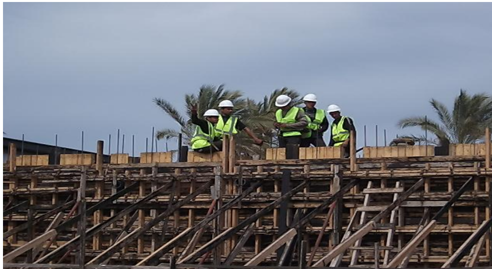
Figure 12. Construction of Seawater Reservoir in Deir Al Balah RO Desalination Plant
