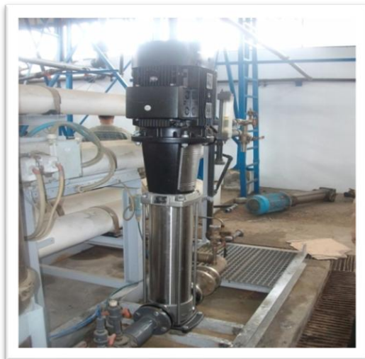
Figure.16- Repair of a High Pressure Pump
