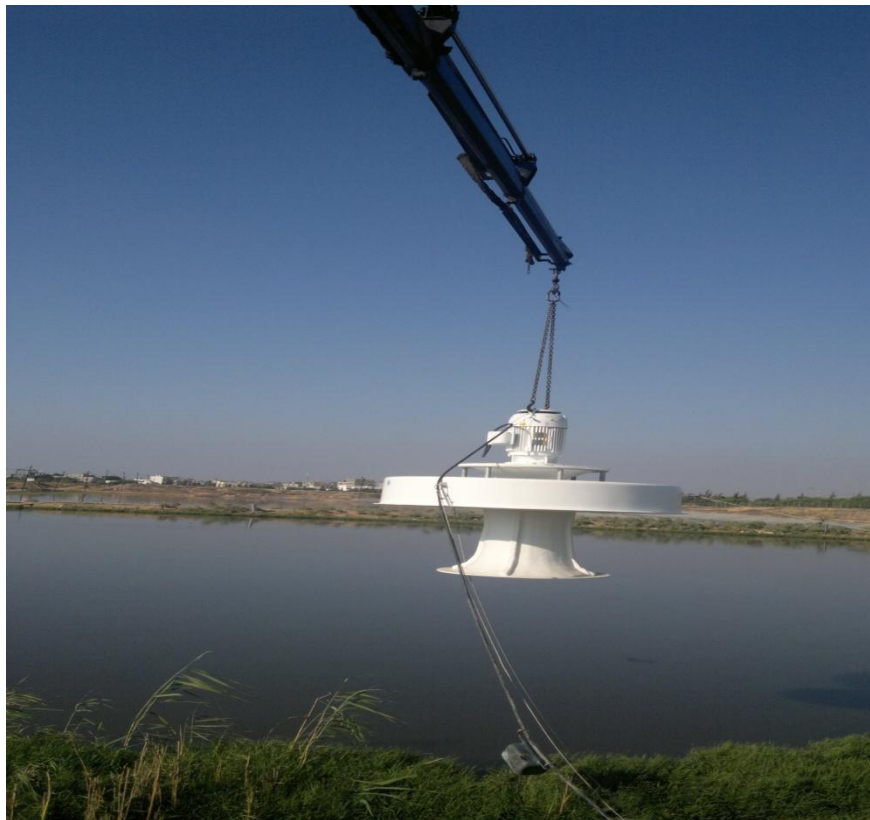
Figure. 25 Installation of Mechanical Floating Aerator-BLWWTP
