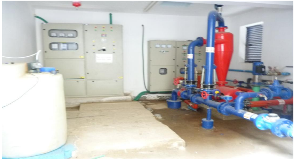
Figure 13- Rehabilitation of Taj Al Waqar Water Well, Al Nussirate
