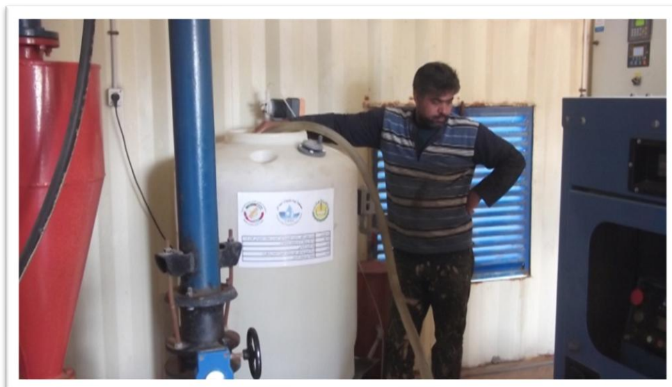
Figure 8-Chlorine Dosing Unit
