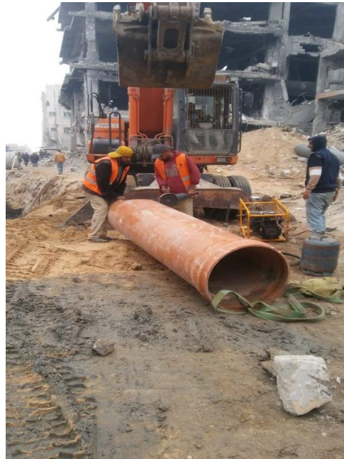
Maintenance of stormwater pipelines at Jamal Abed Al Naser in Khan Younis
