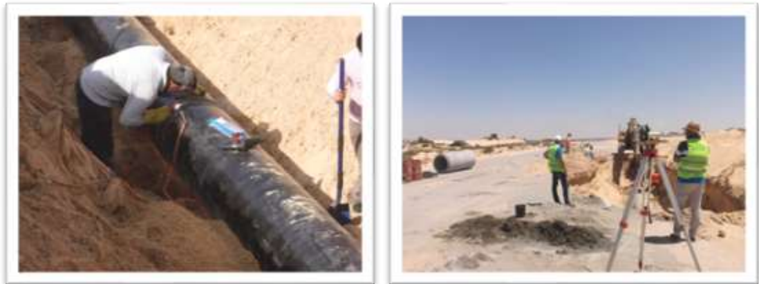
Figure 39: Al Amal Storm Water Project
