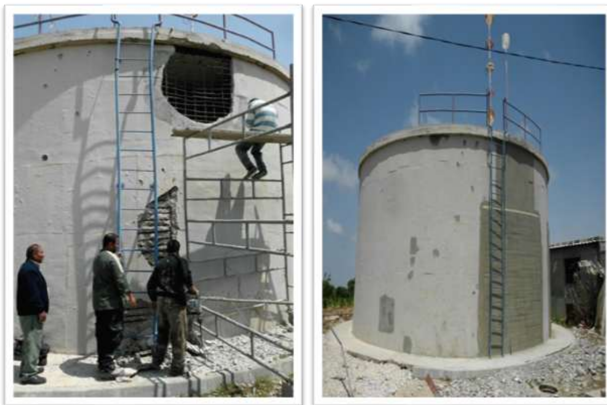
Figure 31: Al Qarara Water Tank
