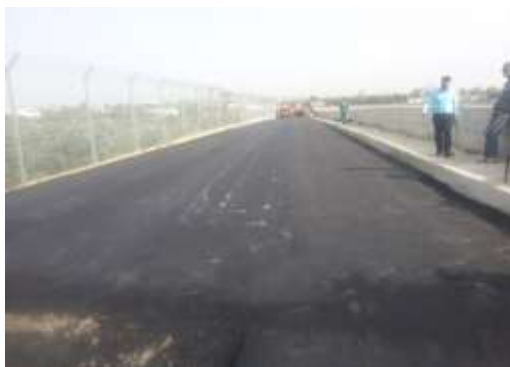
Internal Roads at CWWTW
