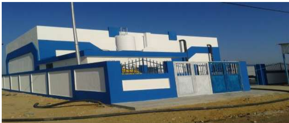
Figure 26: Khuzaa Re-constructed Water Tank
