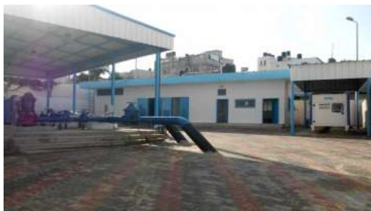
Figure 24: Bani Suhila Water Tank
