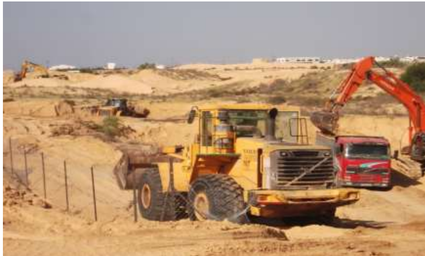
Figure 42: Excavation Rafah Storm water pond
