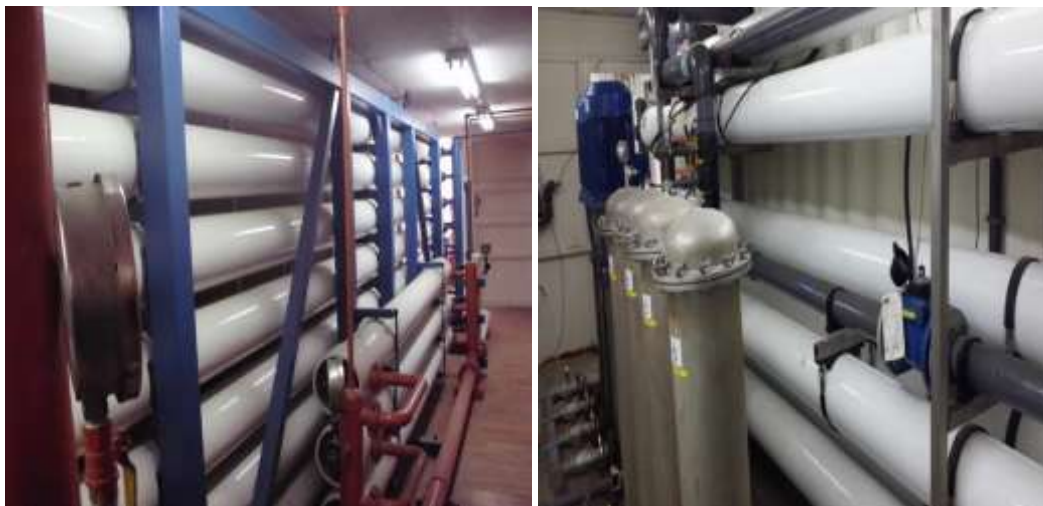
Figure 20: Maintenance work at Deir Al Balah Sea Water Desalination Plant
