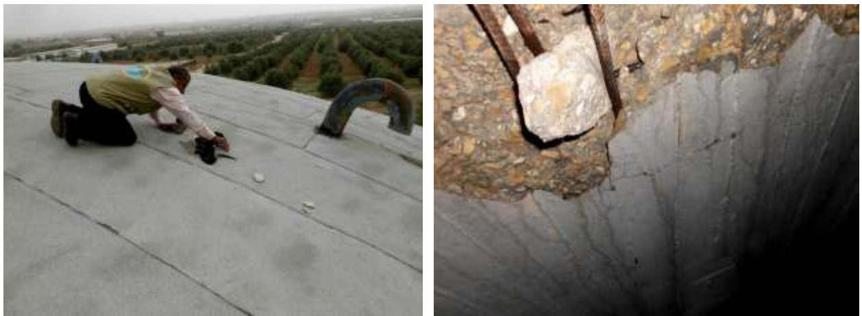
Figure 34: Water Tanks to be repaired in phase II
