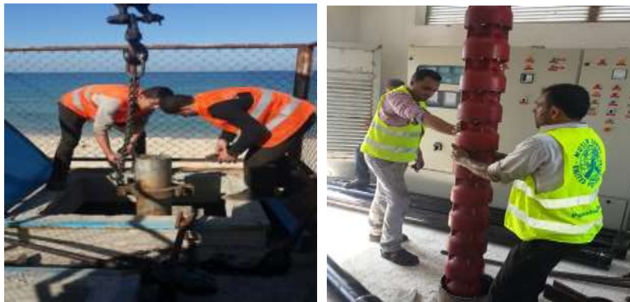
Figure 7: Installation of vertical turbine pump
