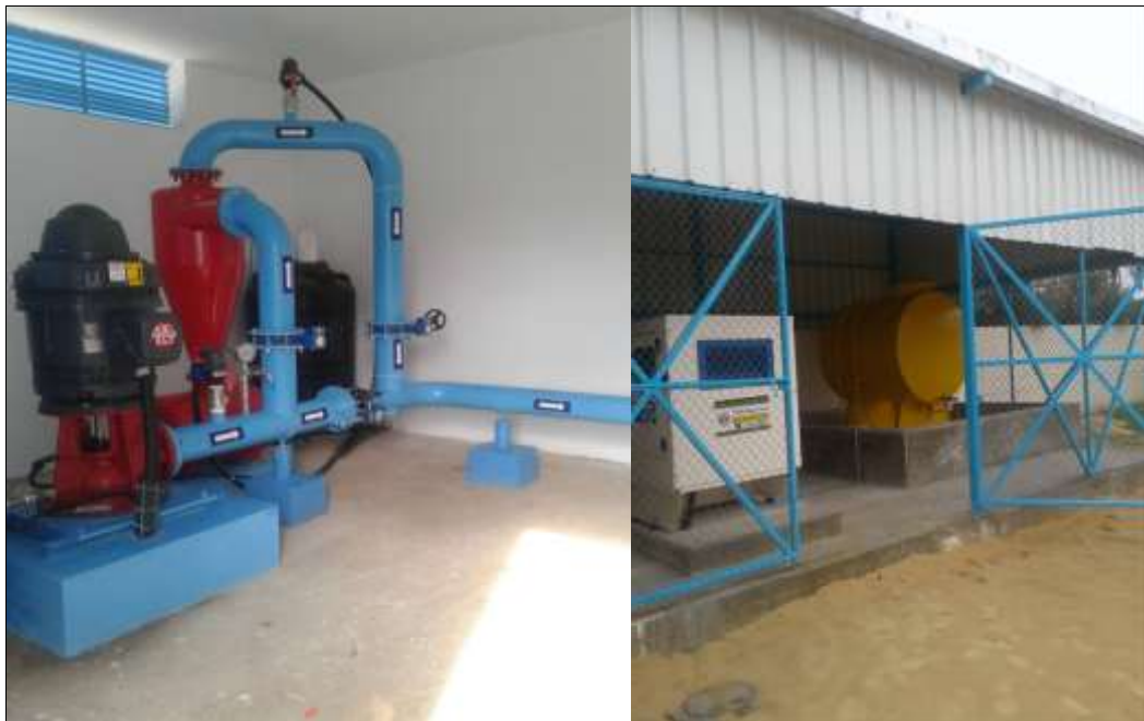
Figure 3 : Drilling and construction of Al Fayrouz new water well in Deir Al Balah
