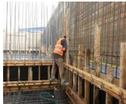
Muntar Water Tank
