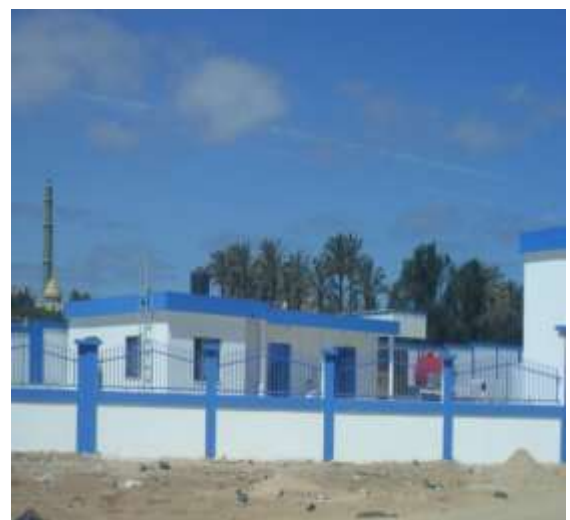
Figure 43: Al Nussirat Sewage Pumping Station
