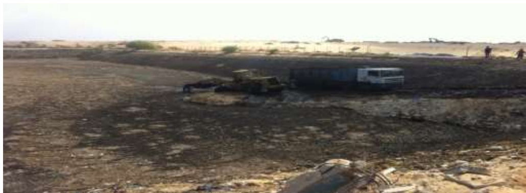
Figure 37: Cleaning Lagoon No. 1 in Khanyounis Temporary WWTP
