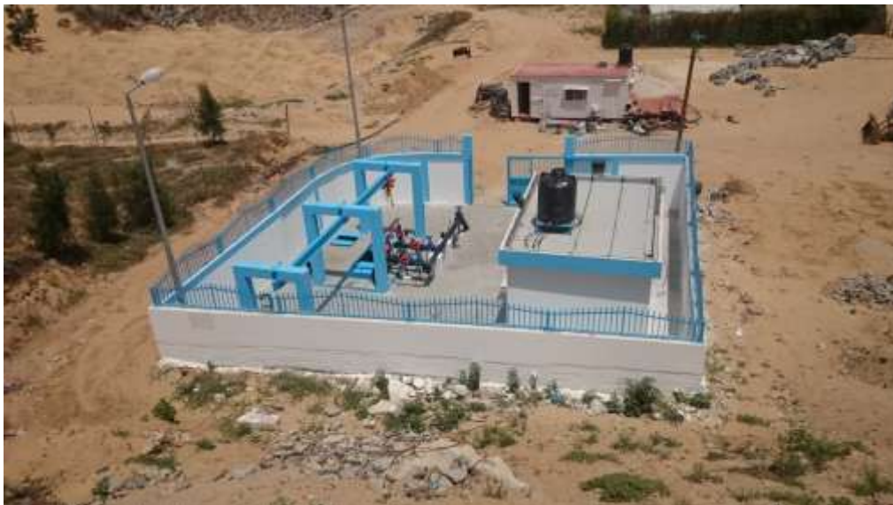
Figure 45: Baten El Sameen sewage pump station in Khanyounis
